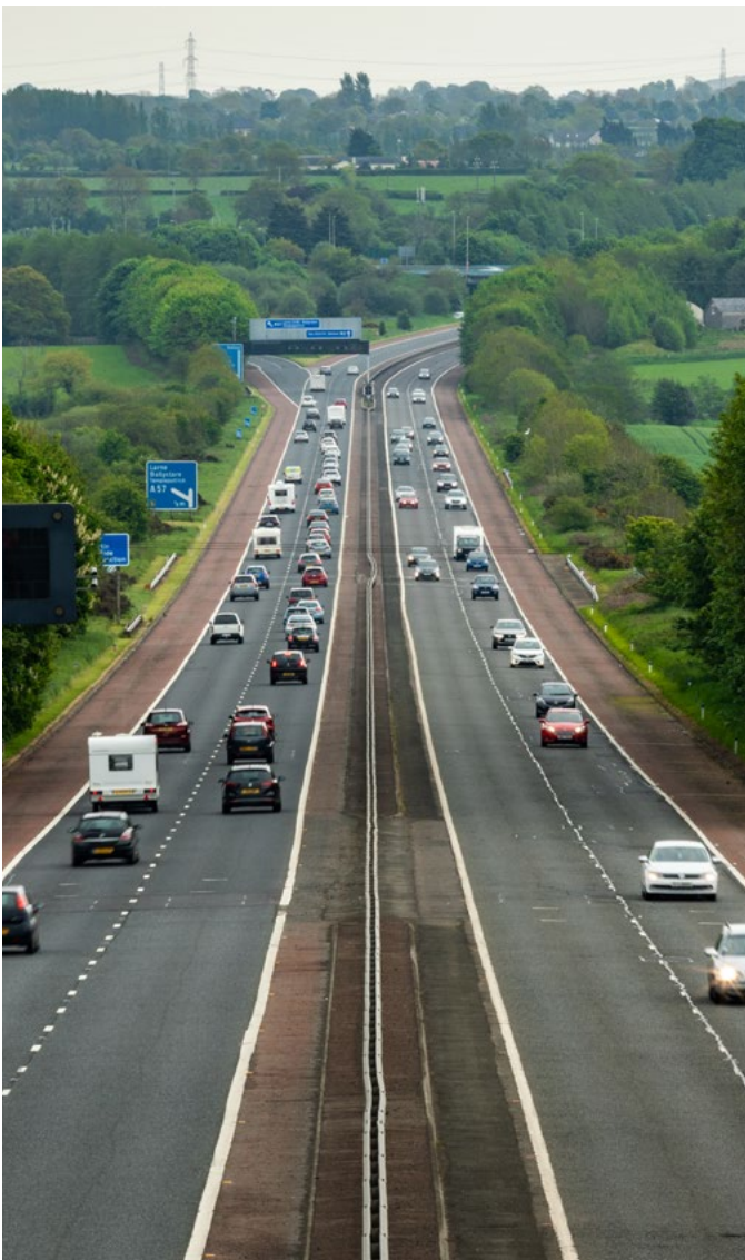
M2 Motorway, Northern Ireland
