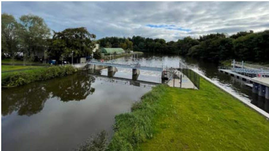
The refurbished Stranmillis Weir in operation.
