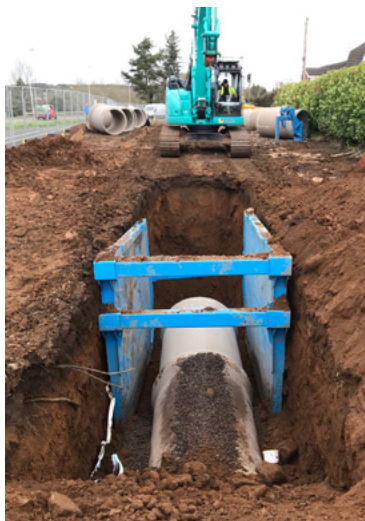
A new 1200mm concrete pipe being installed as part of the FAS in the Prince William Road area of Lisburn. This larger pipe will increase the capacity of the drainage network, helping to alleviate flooding issues in this area of Lisburn.
