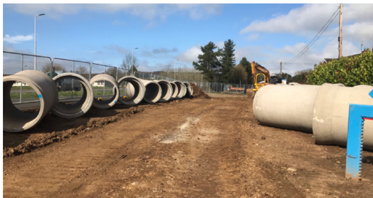
A new 1200mm concrete pipe being installed as part of the FAS in the Prince William Road area of Lisburn. This larger pipe will increase the capacity of the drainage network, helping to alleviate flooding issues in this area of Lisburn.
