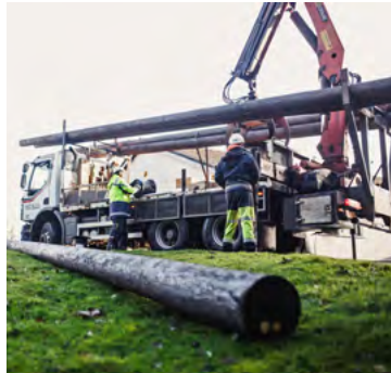
Replacing downed electricity poles
