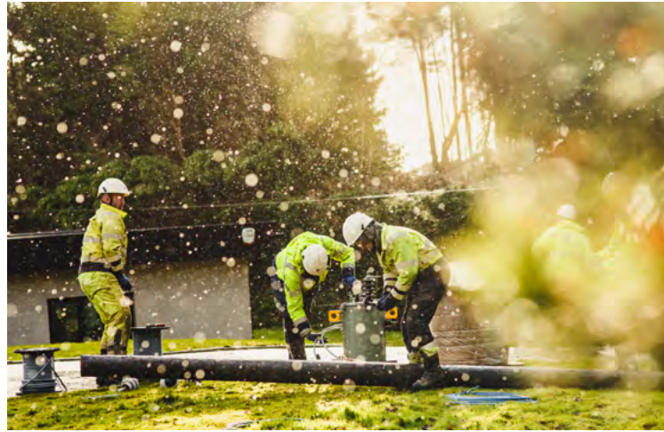
An NIE Networks crew works to repair a damaged power line
