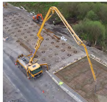
Concrete is poured to create a slab on the supporting piles
