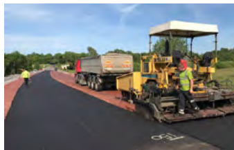
Resurfacing the new raised section of the B127
