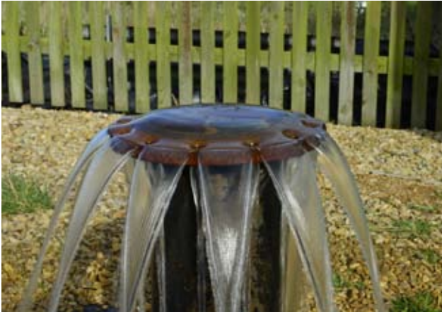
An artesian borehole.
