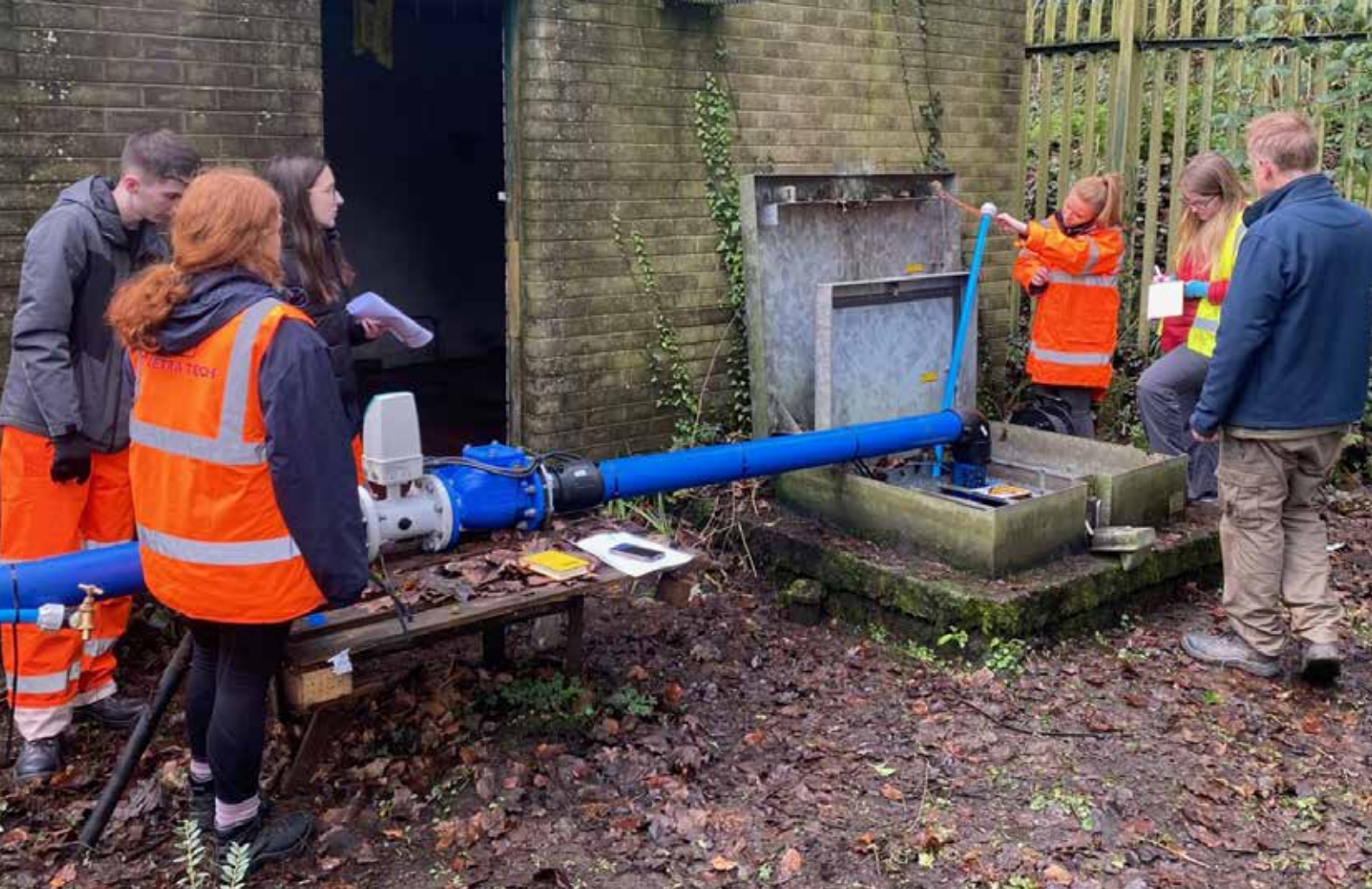
GSNI visiting an NI Water pumping test as part of work delivered through the NI Water SLA.
