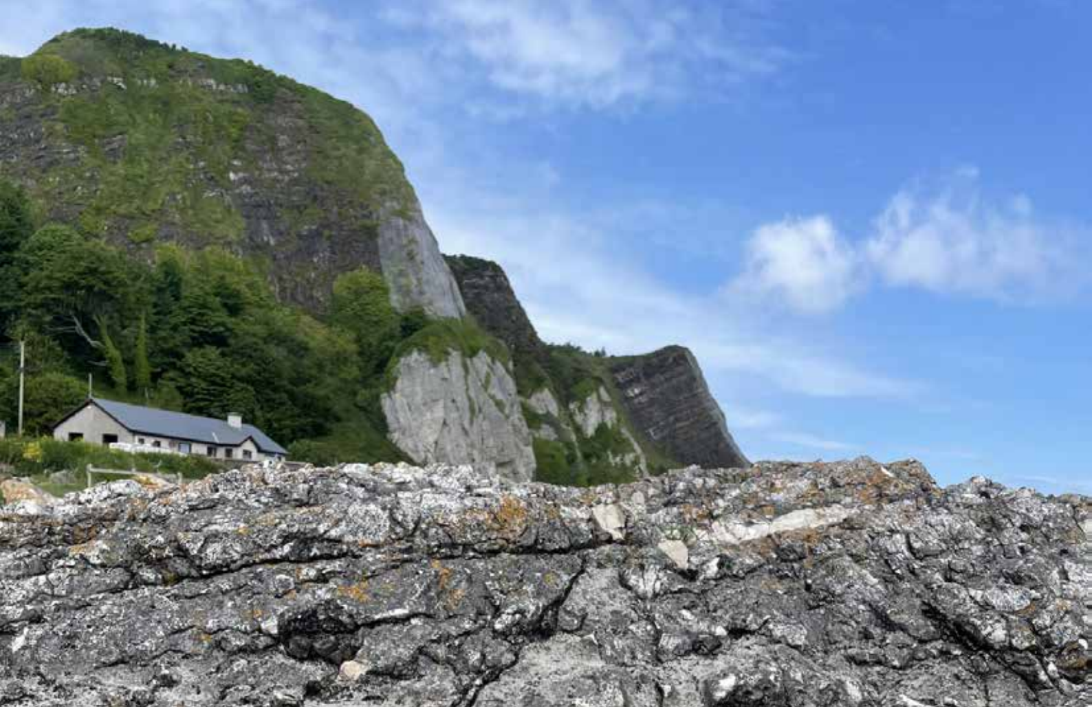
The Garron Point landslide.
