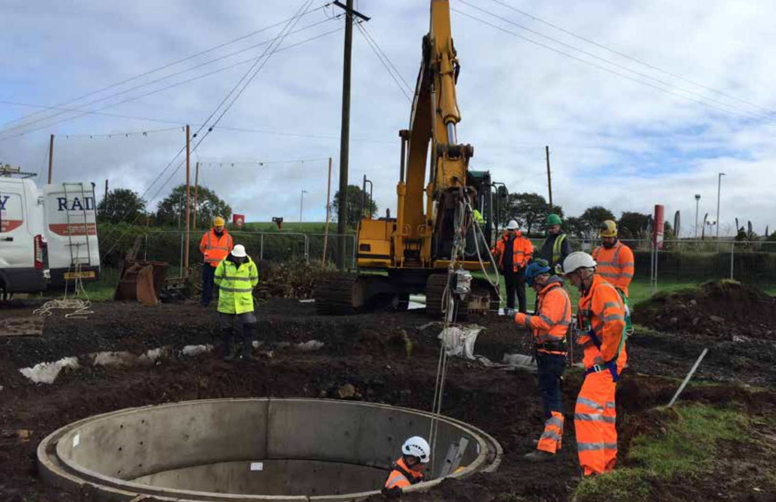
Underground investigations at Rathkenny as part of the abandoned mine programme
