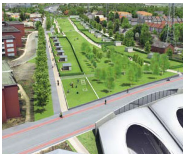
Figure 21. Decking over the A7 autobahn, Hamburg.
