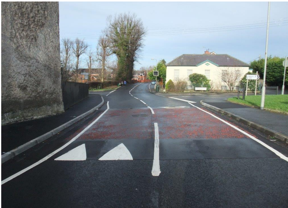
Lower Ballinderry Village, Lisburn (After)
