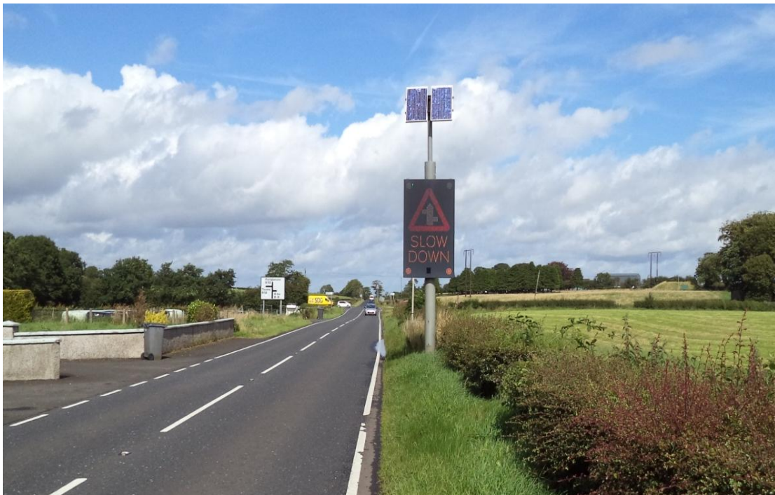
Fig. 5: Speed Reactive Junction Warning Signs at Kilknock Cross, Largy Road.
