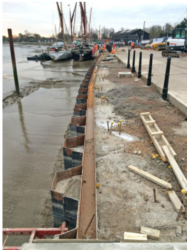
Figure 2-8 - Backfill behind a sheet pile wall
