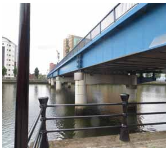
Plate 4.1 – Lagan Railway Bridge crossing the downstream section of the Impoundment.
