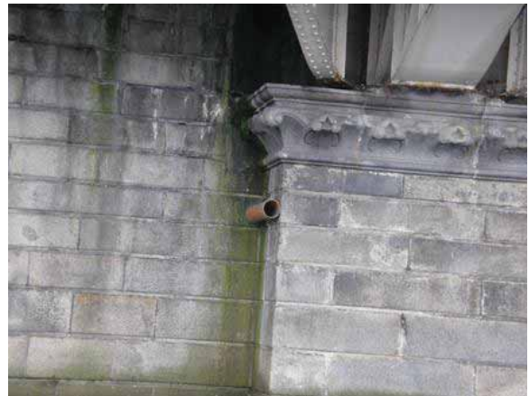
Plate 4.11 – Guillemot nesting tube installed by DSD staff on Queens Bridge.
