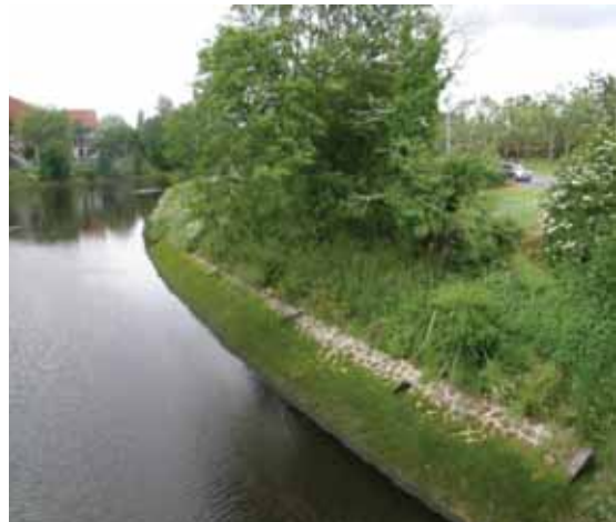
Plate 3.2 – Hard engineered riparian edge upstream of Governor's Bridge, showing revetment, narrow grassland strip and tree/shrub at the top.
