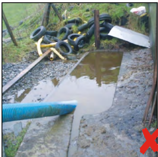
Photo 12 - Overflowing effluent tank not being managed
