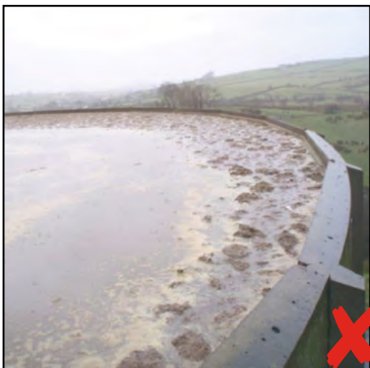
Photo 10 - Freeboard on above ground slurry tank not being maintained
