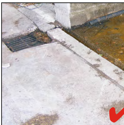
Photo 13 - Silage clamp with well maintained channels draining to effluent tank
