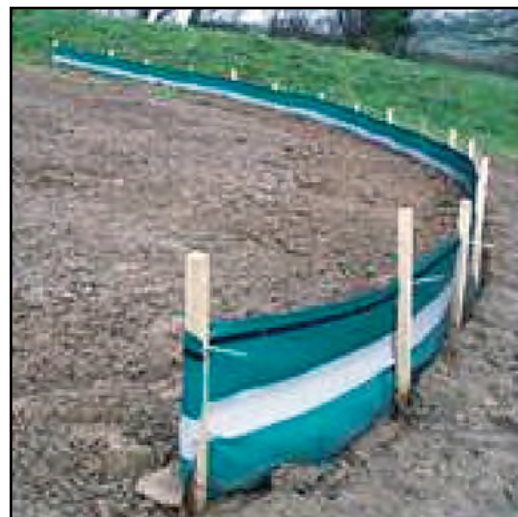
Photo 22 - Sediment fencing
