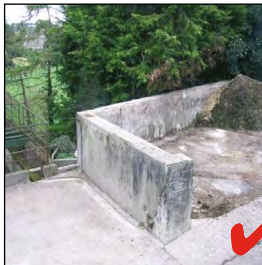
Photo 15 - Midden with all manure contained and run-off collected
