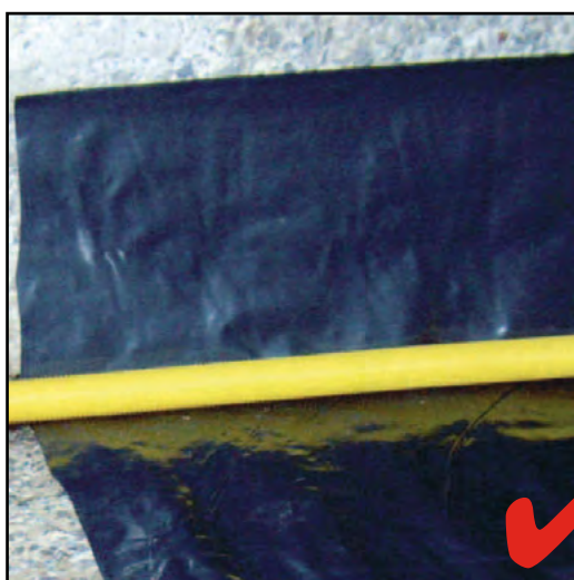
Photo 9 - Protecting silage pit wall-floor joints
