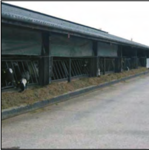
Photo 30 - Yard producing clean water.
