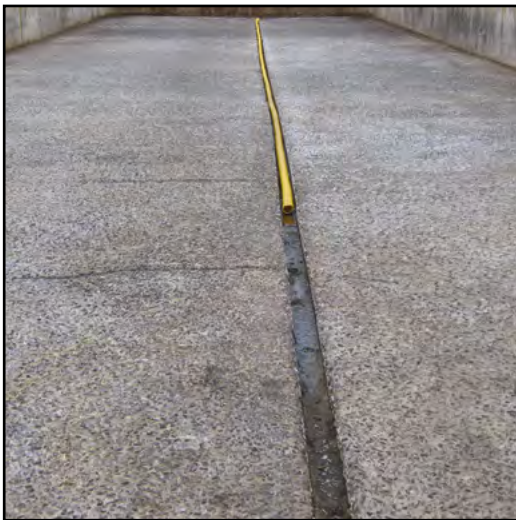
Photo 32 - Run-off from an empty and cleaned silo would be clean water.
