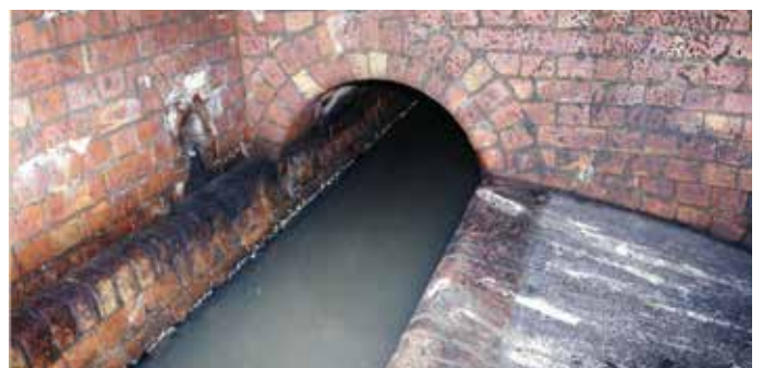
Figure 3.9 – Original Brick Combined Sewer Overflow Chamber
