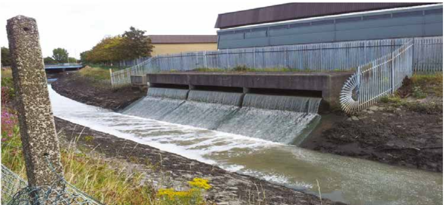
Figure 4.11 - Emergency Overflow at Sydenham WwPS
