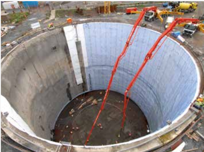
Figure 3: The Tunnel Pumping Station Shaft under construction
