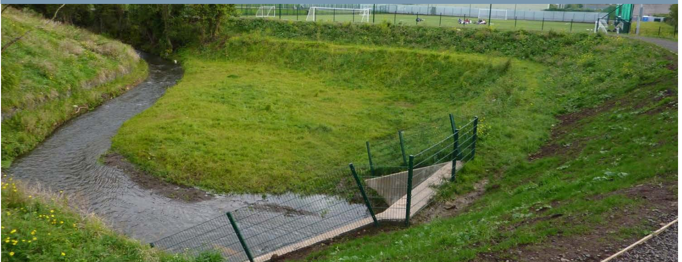
Figure 5.11-9: Sullatober Water Flood Alleviation Scheme storage pond in Shaftesbury Park
