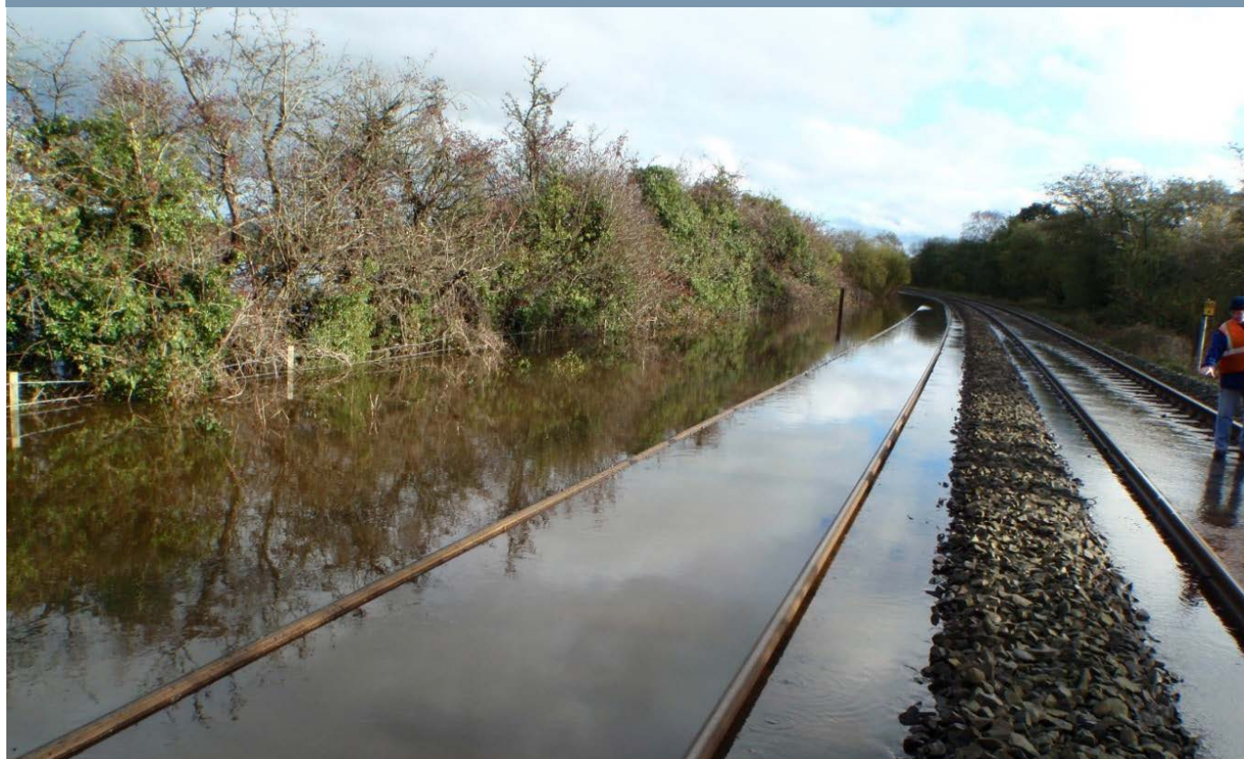
Figure 5.8-2: Flooding of the North/South railway line to the south of Portadown, October 2011
