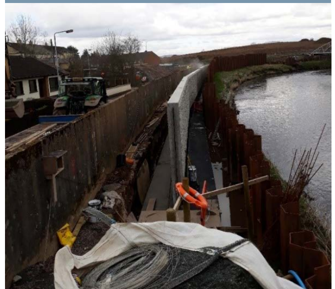
Figure 5.9-13: Floodwall construction as part of the Hunter Crescent Flood Defence scheme
