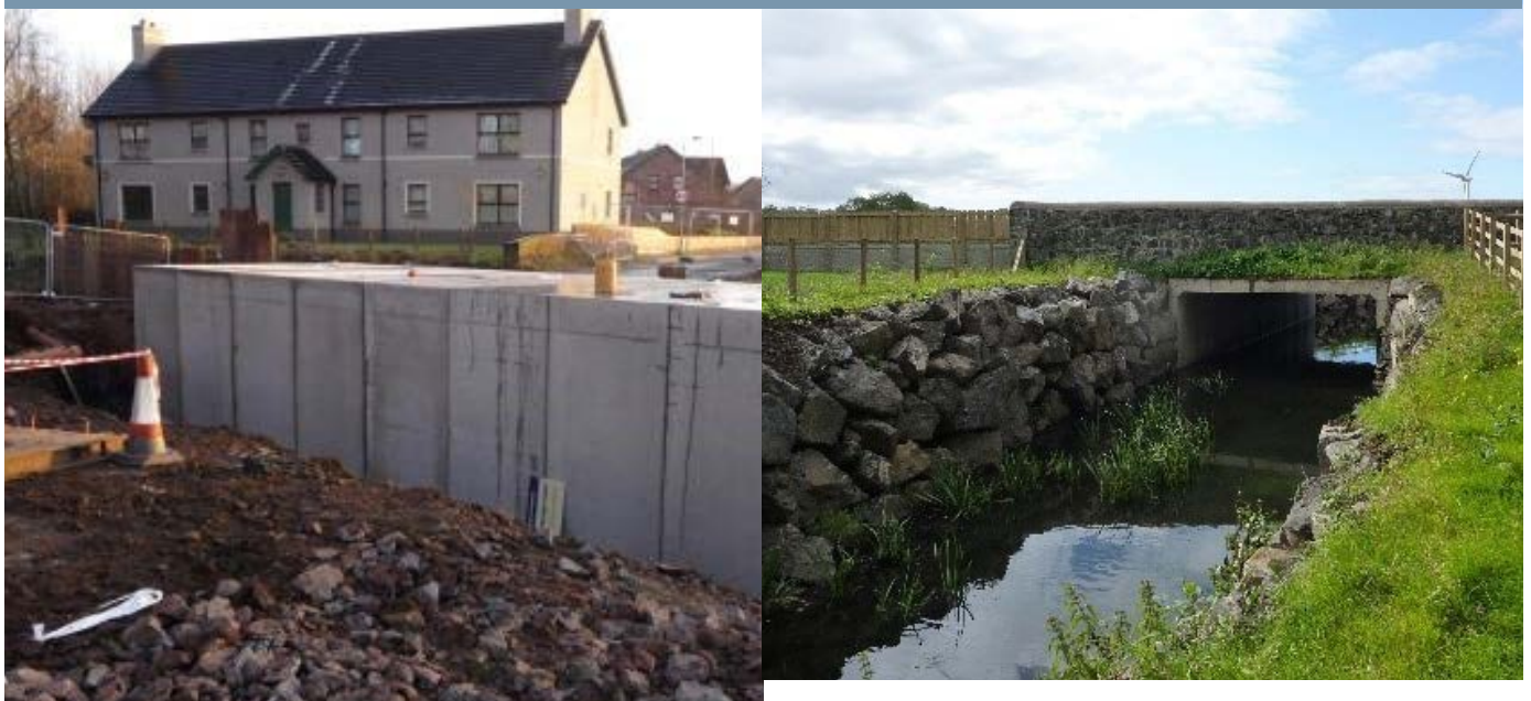
Figure 5.5-10: Photographs taken during Park Road culvert construction and of completed works
