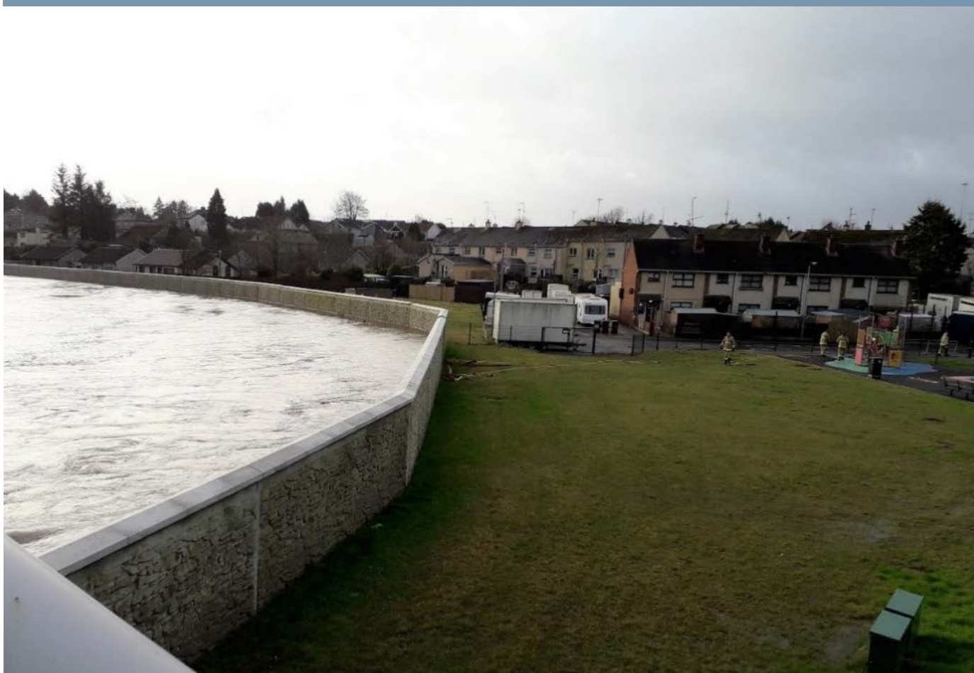
Figure 5.9-12: Hunter Crescent Defences during a flood in February 2020
