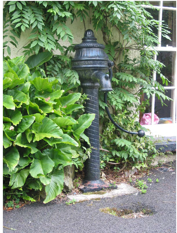
Typical private water pump, Castledawson (HB08/10/005C, Grade B1)
