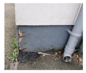
The existing prefabricated buildings are in an increasingly poor state. There are holes in walls, roof leaks (including around electrics and fuse boxes) and general structural issues across the whole school. In many instances, there are issues surrounding bases of the mobiles and there have been several issues with rodents gaining access to them as a result. Additionally, recent work contracted by the Education Authority saw painting and protection of the mobiles incomplete.
