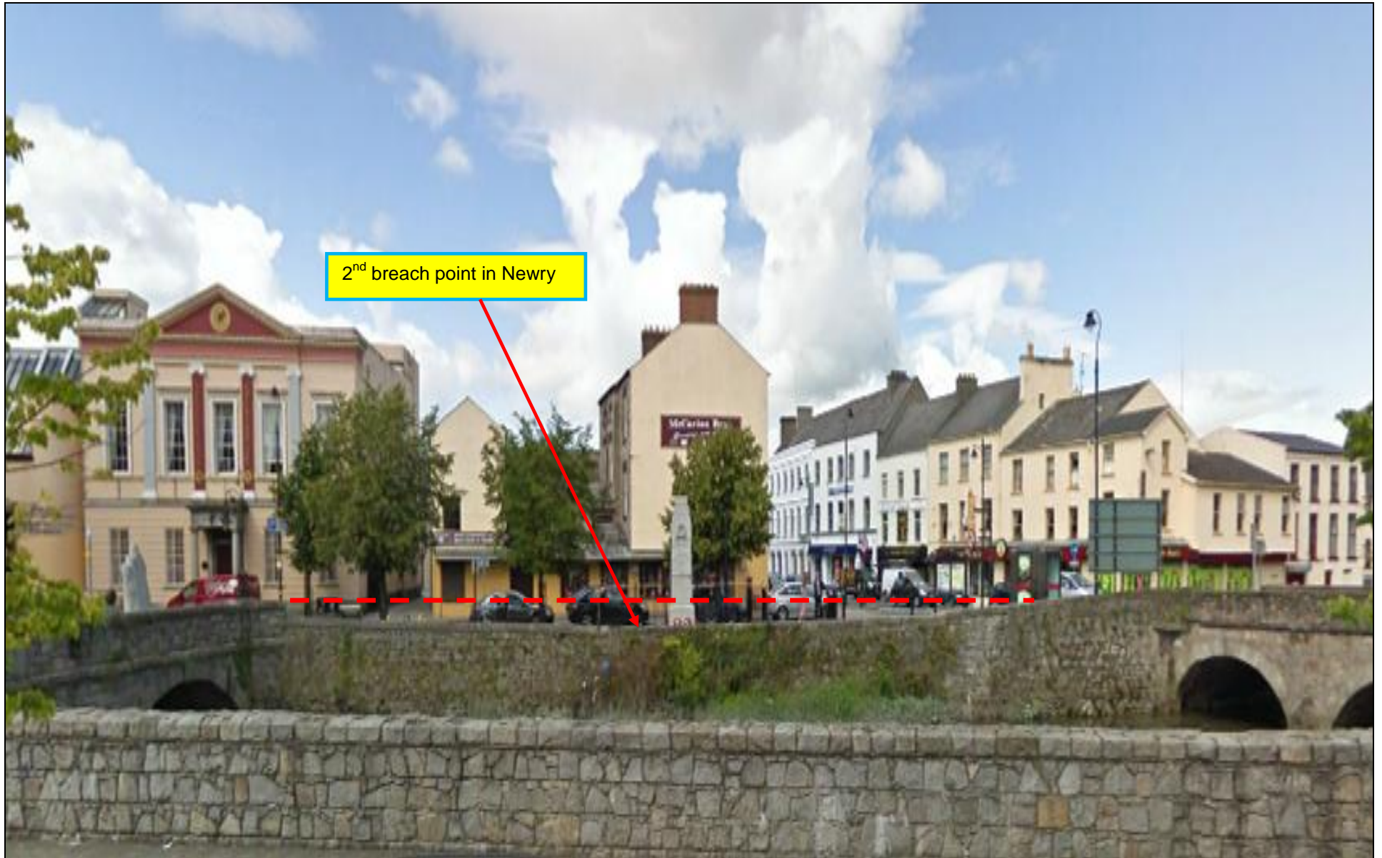
Photo 5.6.6.1 - Second breach point in Newry – Upstream of Newry Town Hall at the War Memorial
