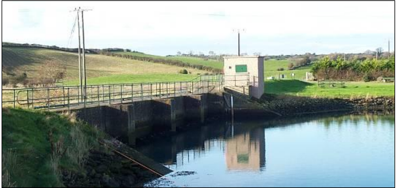
Photo 7.4.3.1 - Quoile Barrier (sea facing aspect)
