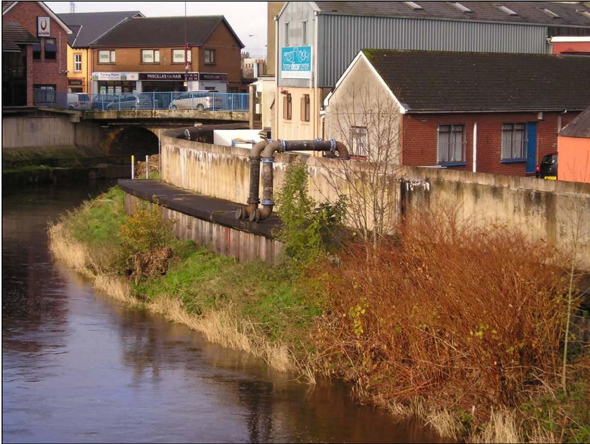
Photograph 6.3.1 – Upstream of Campsie Bridge on the Drumragh River
