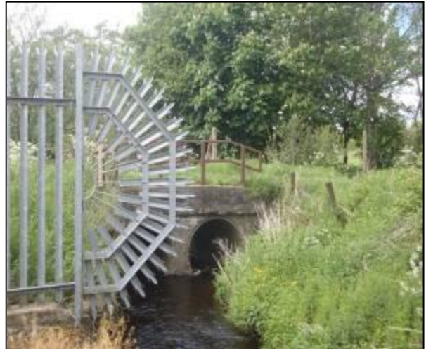
Photo 5.5.4.1 Twin 1500mm dia foot bridge on Ballee Burn
