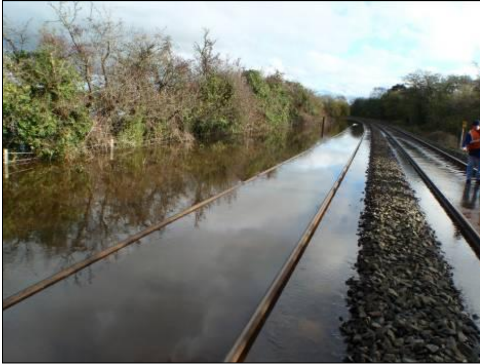
Photo 5.8.2.1 - Portadown Railway line flooded in Oct 2011
