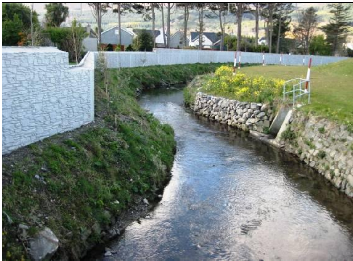
Photograph 7.7.1.1 - Newcastle, Burren River flood defences.
