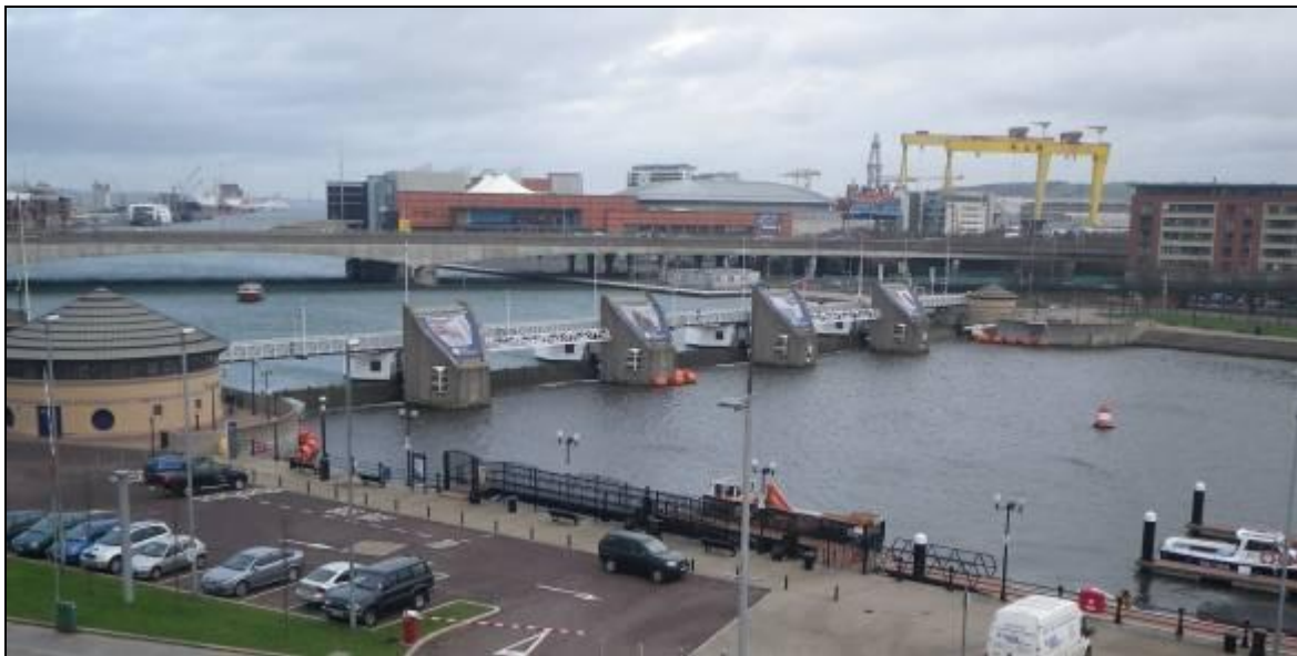
Figure 7.3.1.4 - Belfast SFRA – Lagan Weir
