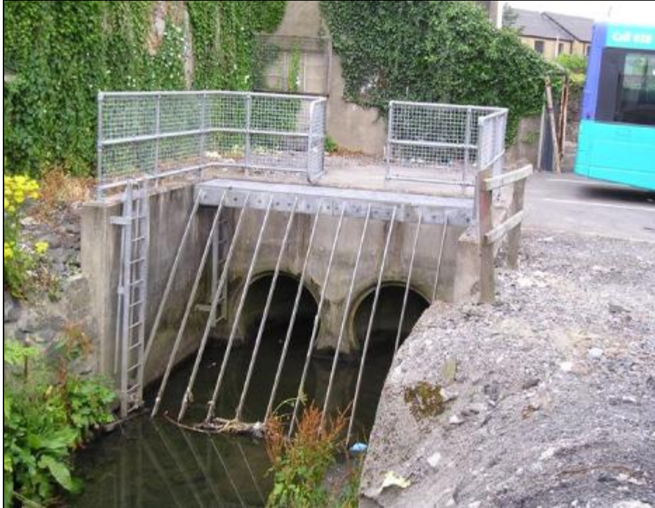
Photo 5.6.1.5 - Inlet Structure on Derrybeg River
