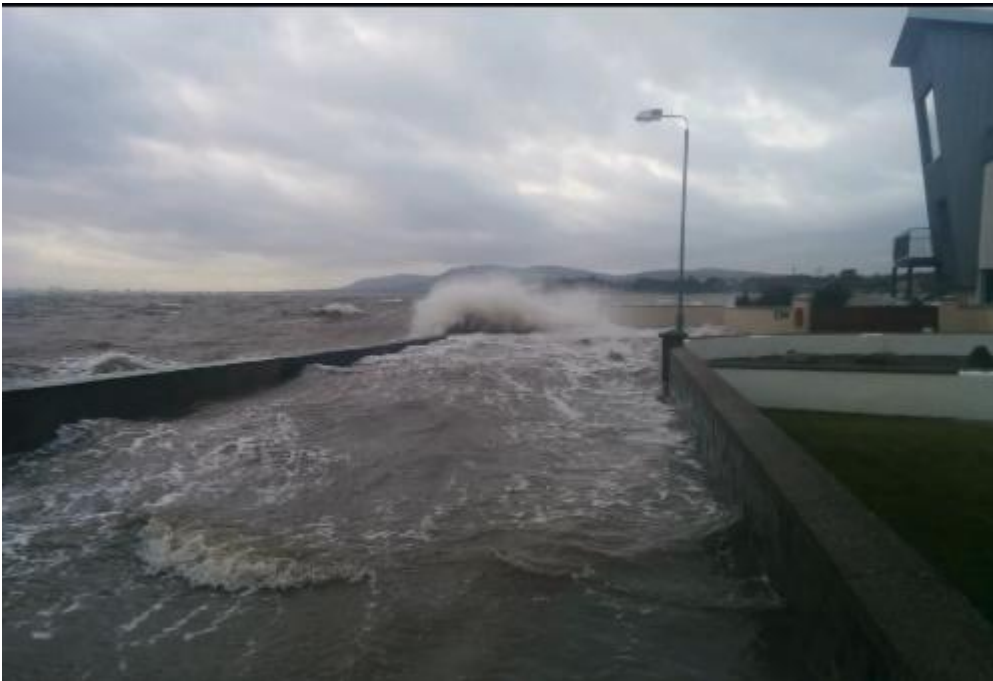
Photograph 7.9.1.1 - Carrickfergus Coastal Flooding – 3 January 2014
