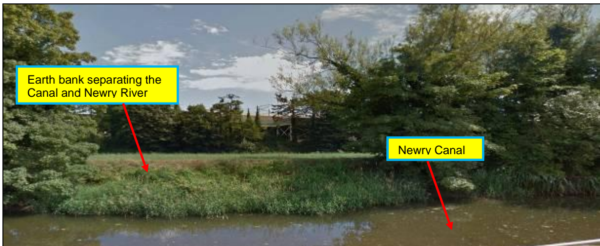
Photo 5.6.1.4 - Earth flood bank that separates the Newry Canal and the Newry River that was raised in 2001
