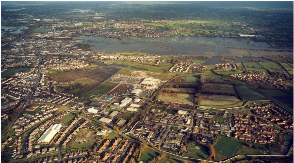
Figure 5.8.2.1 - Flooding in Portadown 2000
