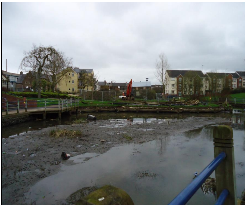
Photo 5.11.1.1 – Anderson Park pre Flood Alleviation Scheme
