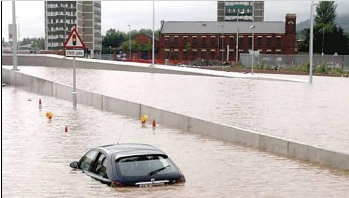
Photograph 7.3.1.2 - Flooding of West Link (Broadway Underpass), 16 August 2008
