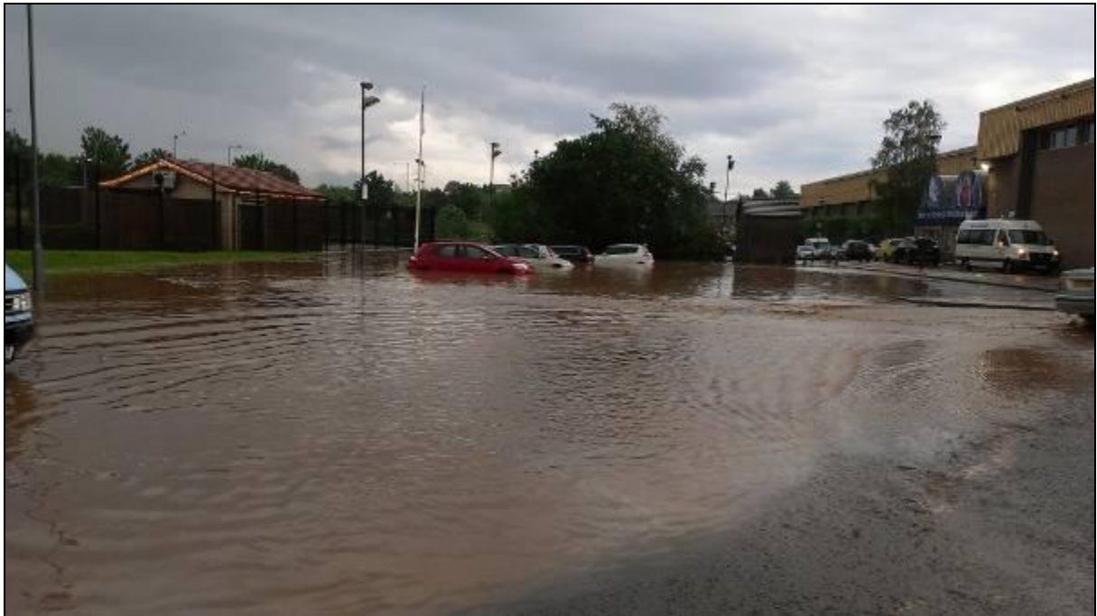
Figure 7.5.1.1 - Flooding at Dundonald Ice Bowl, 27 June 2012
