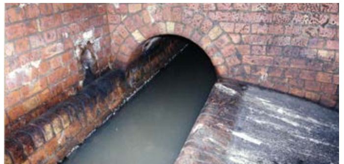
Figure 3.9 – Original Brick Combined Sewer Overflow Chamber
