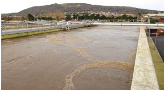
Figure 3.15 – Aeration Lanes at Whitehouse WwTW
