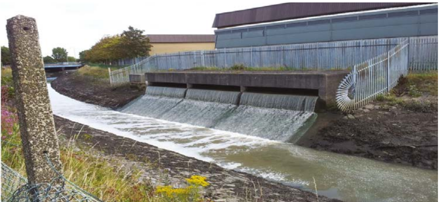
Figure 4.11 - Emergency Overflow at Sydenham WwPS
