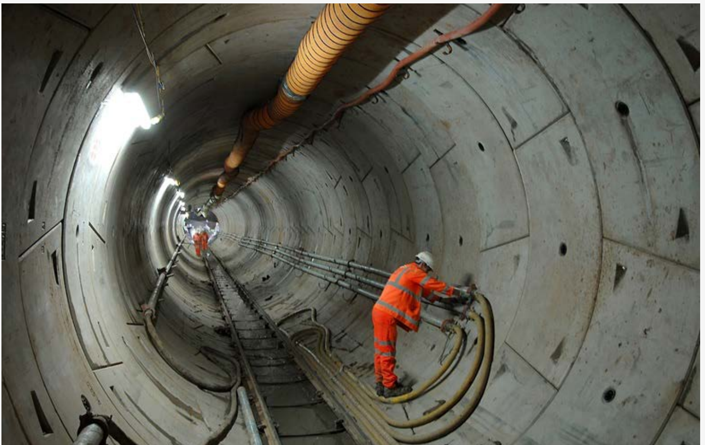
Figure 1: Belfast Storm Tunnel under Construction
