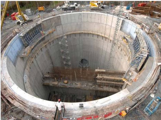
Figure 3: The Tunnel Pumping Station Shaft under construction
