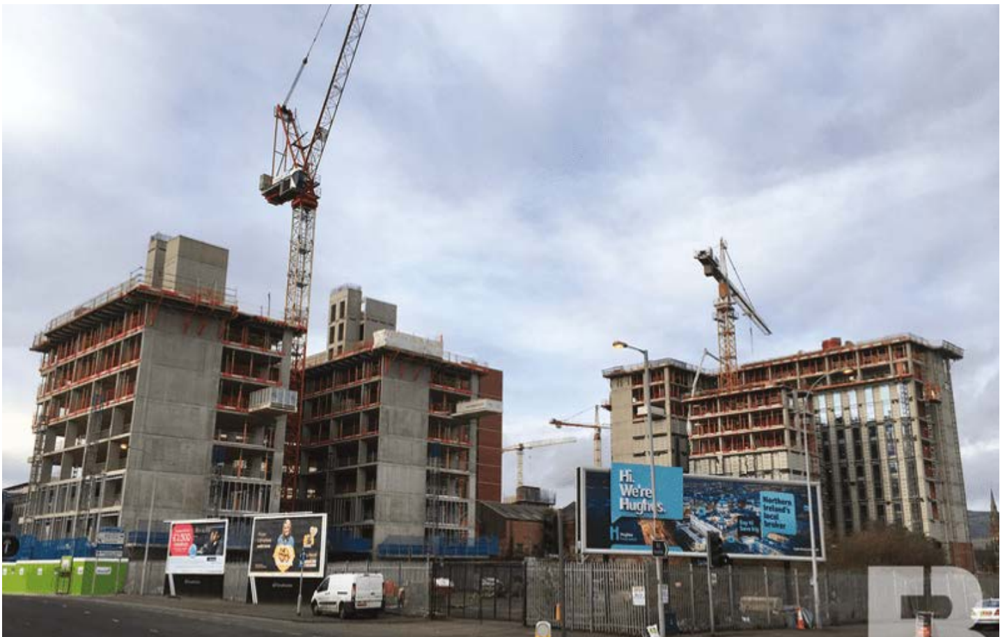
Figure 4.14 - New Ulster University Belfast Campus under construction
