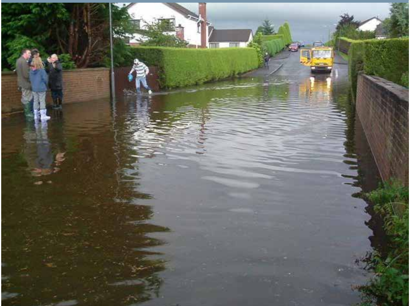
Figure 5.4-2: Flooding at Shane Park, Lurgan, August 2008
