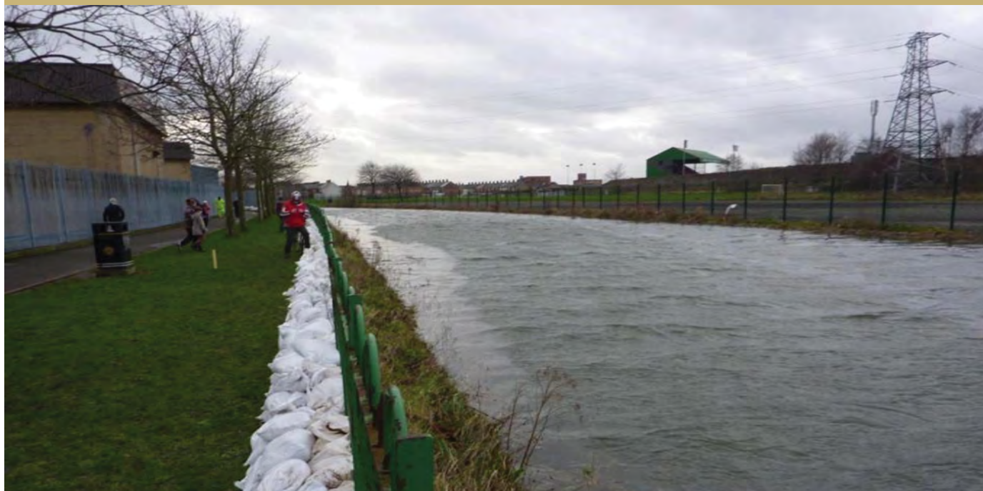
Figure 2-3: Emergency Sand Bag Flood Protection on the Connswater at Sydenham - January 2014
