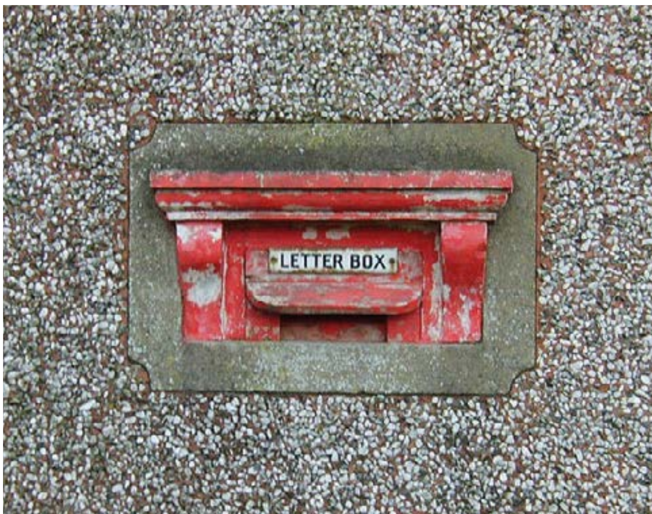
Remnants of timber box at Post Office, Sixmilecross, Omagh
