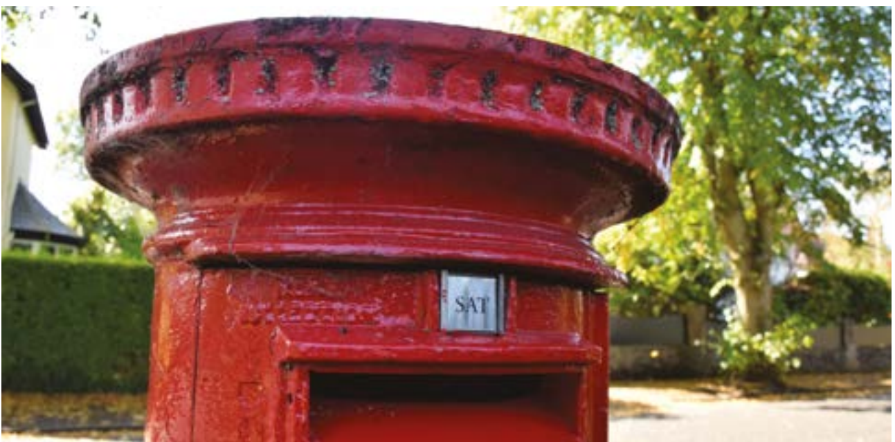
Iconic 'piecrust' flutes feature at the top of pillar boxes to aid water run-off
