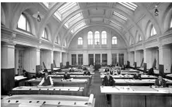
Titanic Drawing offices, Belfast. Historically, natural daylight was the primary source of illumination, and so to maximise light penetration, high windows, high ceilings and a shallow plan depth were designed in to most buildings – both domestic and commercial.
