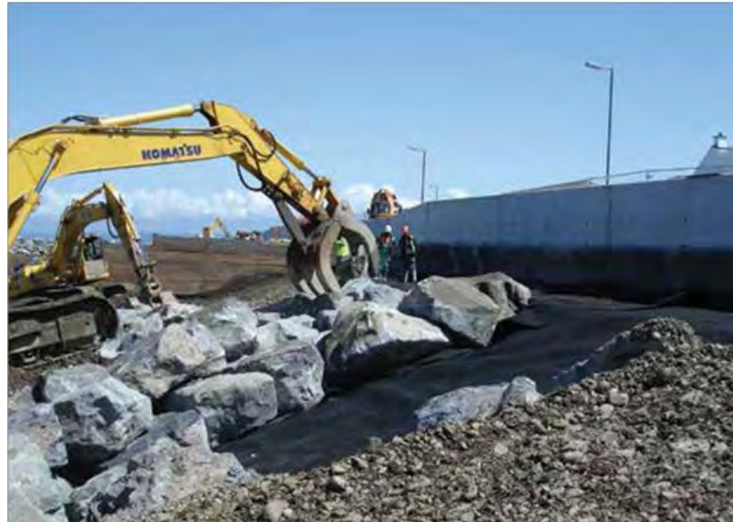
Photograph 5.9: placing rock armour
