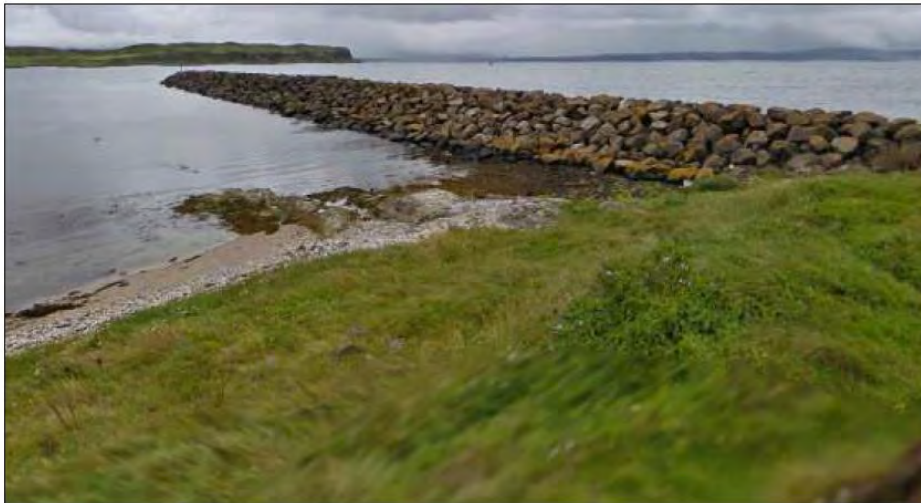
Photograph 7.2: PDA from road at north looking towards south
