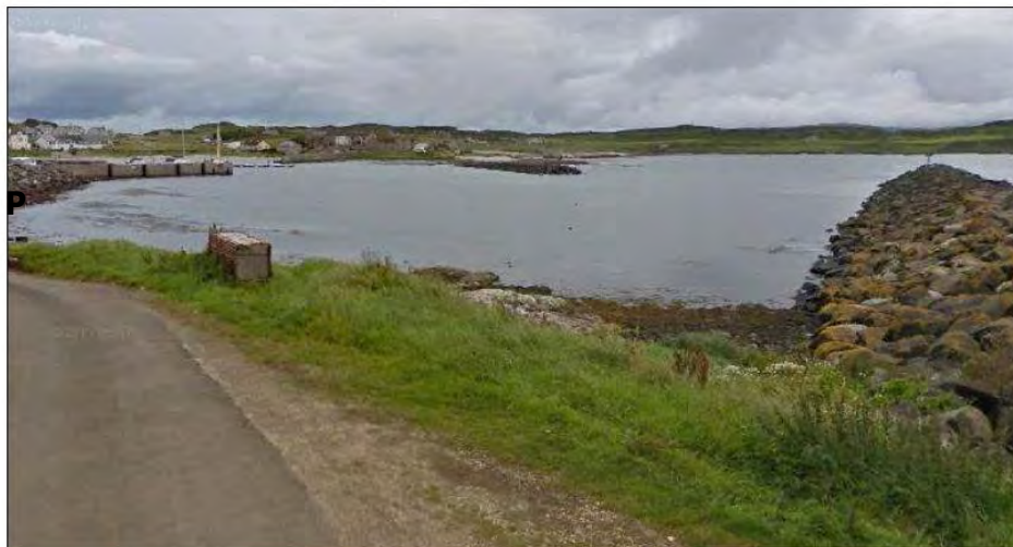
Photograph 7.5: PDA from road at northwest looking towards south-southeast
