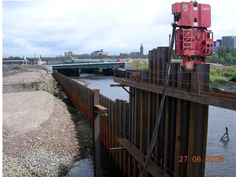
Photograph 5.10: sheet piling
