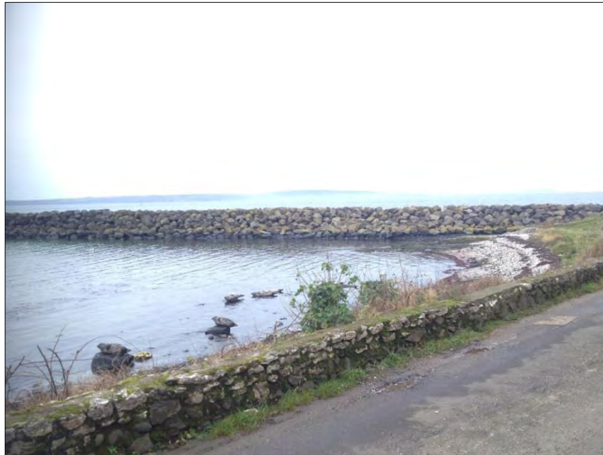
Photograph 4.4: Seals within the proposed area for new slipway
