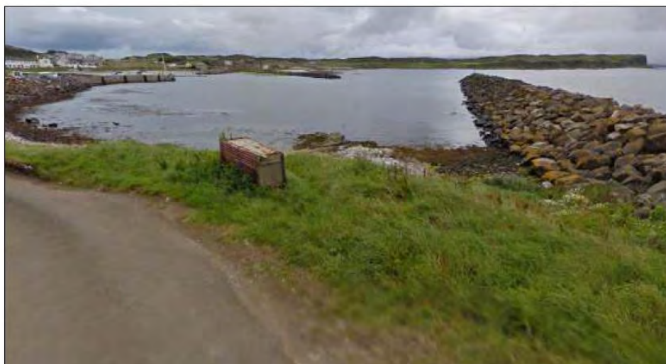
Photograph 7.6: PDA from northwest corner looking towards south
