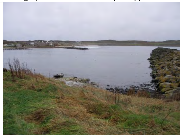
Photograph 5.8: Western breakwater / site of new slipway
