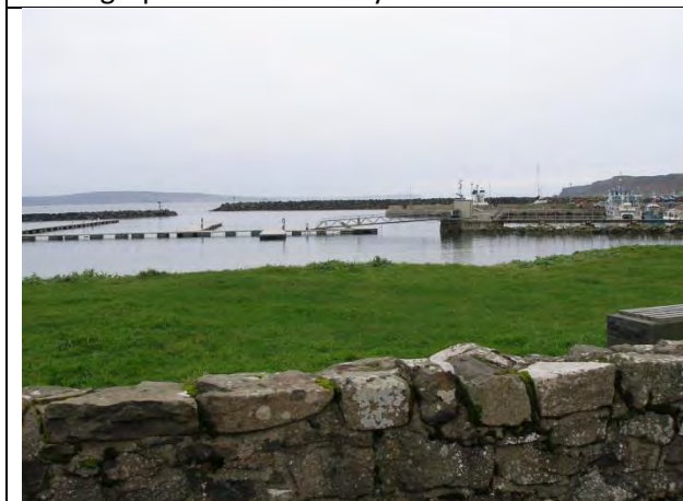
Photograph 5.7: View west over harbour
