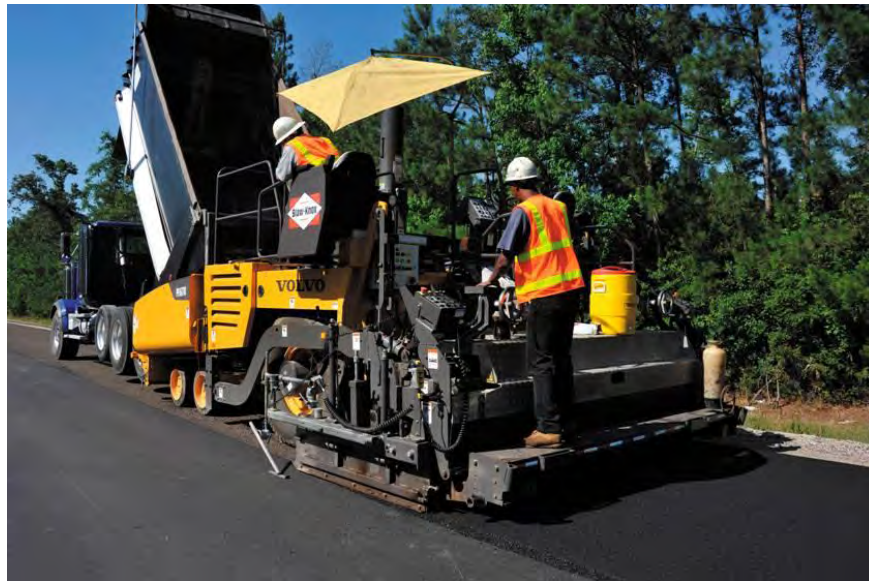
Photograph 5.13: Laying bitmac
