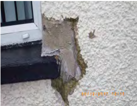
Figure 8.18 Damaged render
