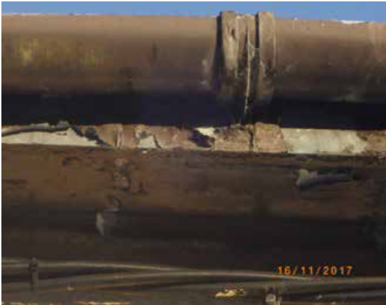
Figure 8.11 Damaged/blocked guttering
