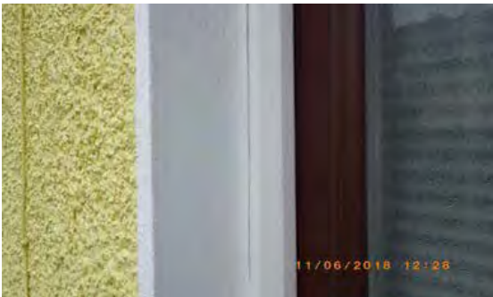
Figure 6.41 Door reveal juncture in a good condition
