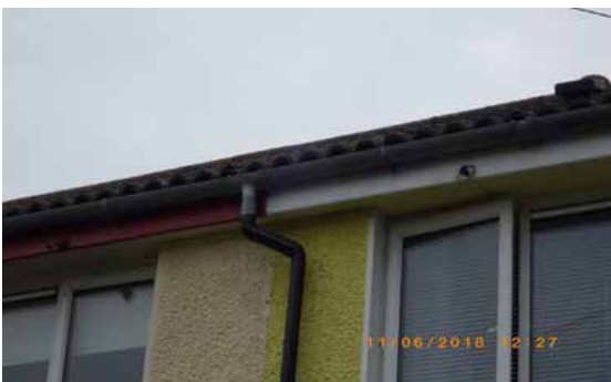
Figure 6.42 Fascia, soffit and guttering in good condition
