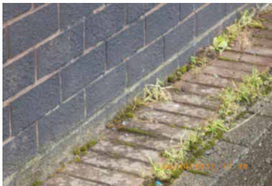
Figure 6.23 DPC below ground level
