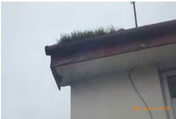
Figure 7.51 Compromised guttering
