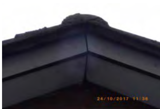
Figure 6.17 Split soffit area
