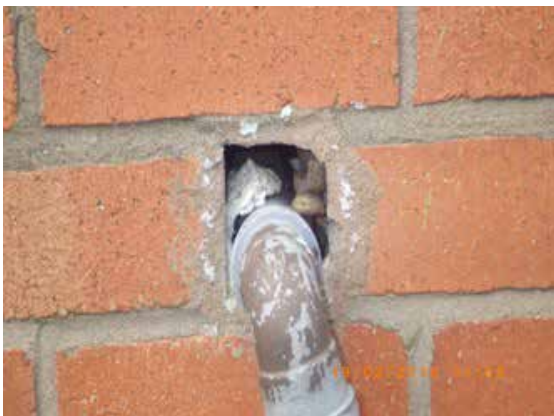
Figure 8.10 Mortar erosion
