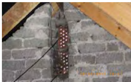
Figure 6.31 Airbrick not sleeved
