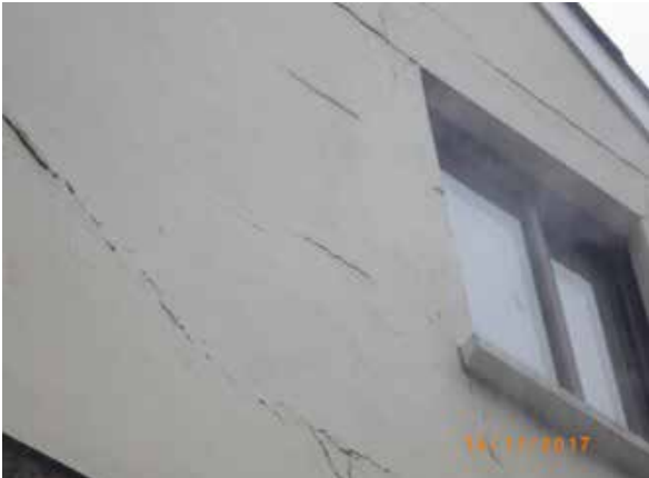
Figure 8.17 Damaged render
