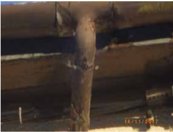
Figure 8.12 Damaged/blocked guttering
