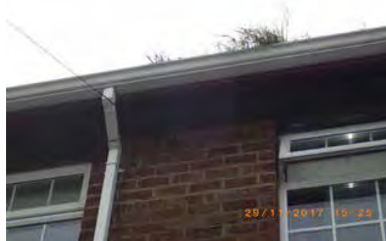
Figure 7.36 Blocked guttering
