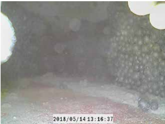
Figure 8.7 Voids in the bead CWI
