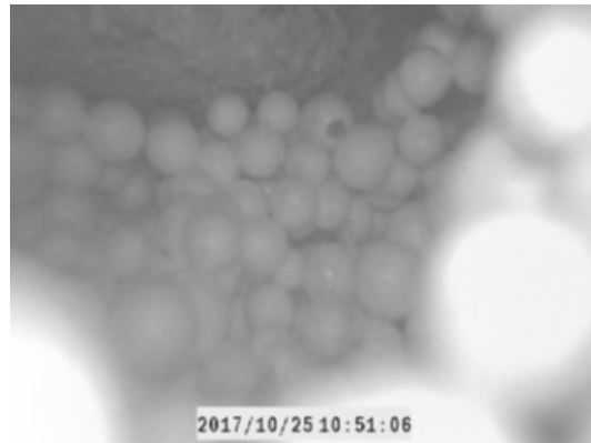
Figure 4.13 Adequacy of CWI fill
