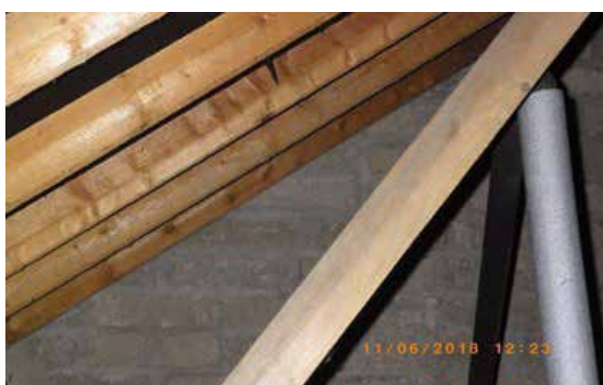
Figure 6.47 Gable wall in good condition
