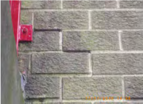
Figure 4.7 Brick and mortar condition
