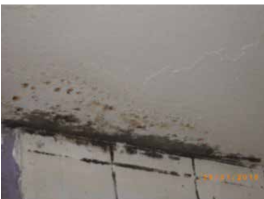
Figure 4.17 Condensation
