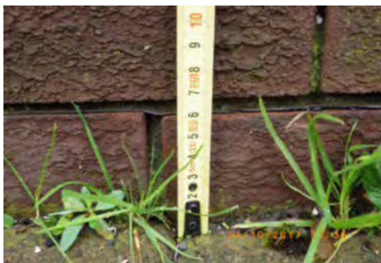
Figure 6.22 DPC level below 60mm
