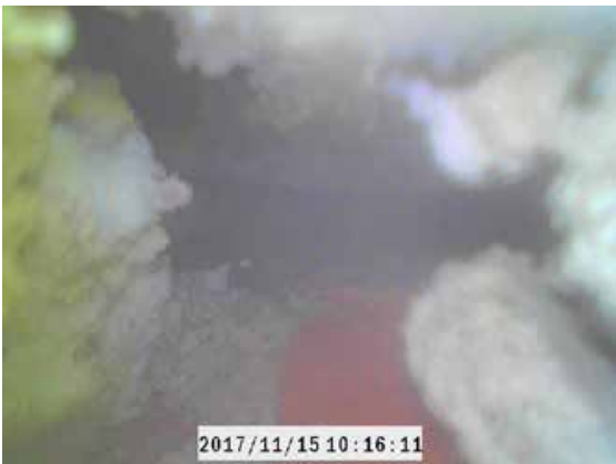
Figure 8.6 Voids and debris in the foam CWI
