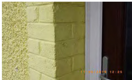
Figure 6.35 Door reveal juncture in good condition
