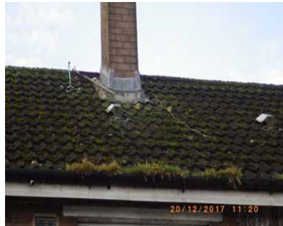
Figure 7.26 Compromised guttering
