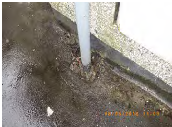
Figure 6.1 Blocked drainage
