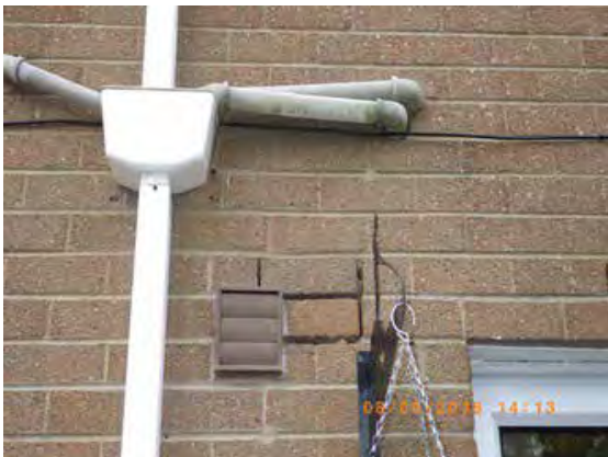
Figure 8.9 Mortar erosion
