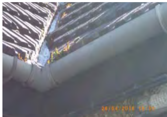
Figure 6.29 Blocked guttering
