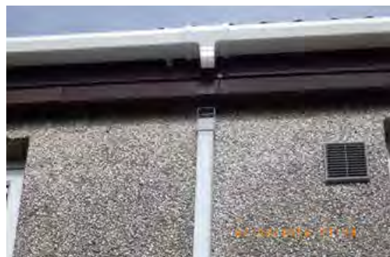
Figure 7.37 Damaged guttering
