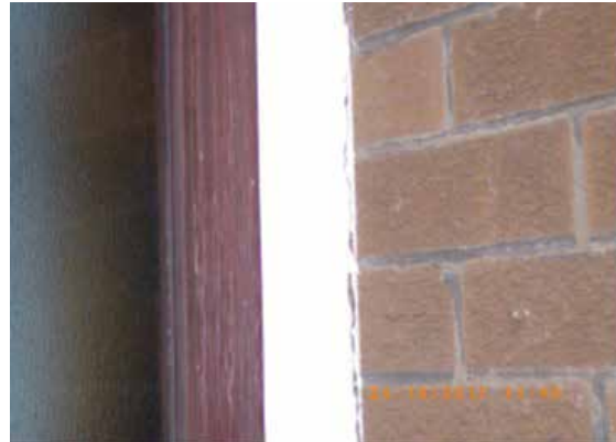
Figure 6.21 Perimeter seals (door)
