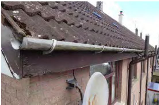
Figure 7.50 Damaged guttering
