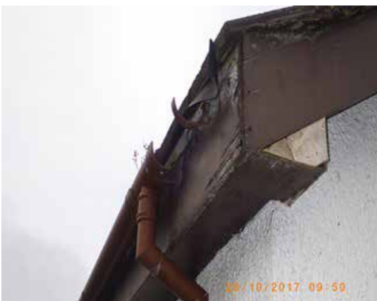
Figure 7.25 Damaged guttering
