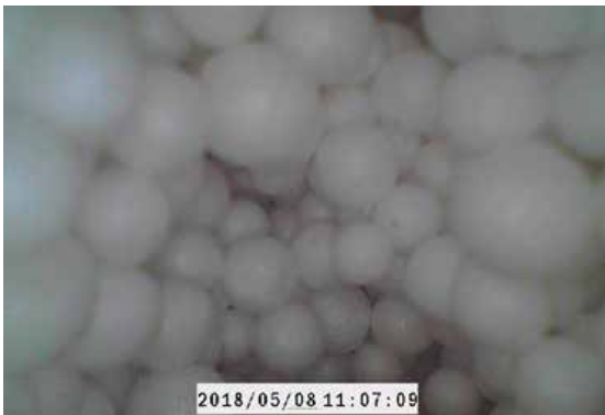
Figure 6.13 Voids in the CWI
