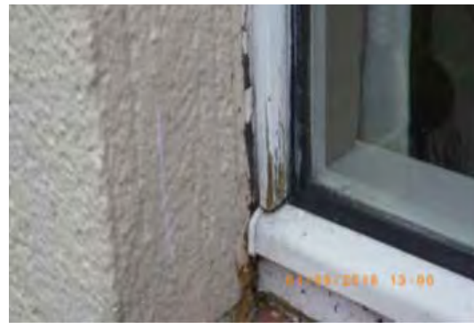
Figure 4.9 Perimeter seal condition (window)
