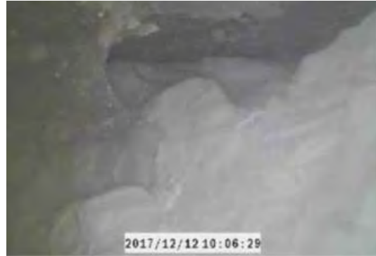
Figure 4.5 CWI System installed
