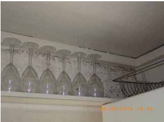
Figure 7.13 Condensation
