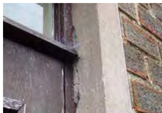
Figure 4.10 Perimeter seal condition (door)
