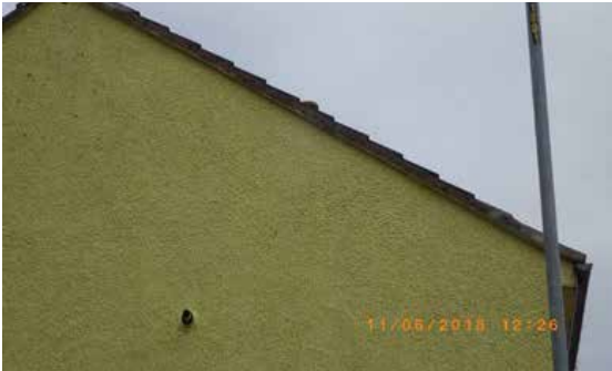
Figure 6.39 Verge edge tiles embedded correctly
