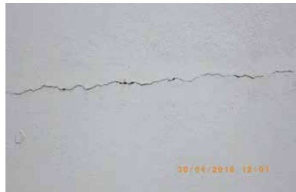
Figure 8.16 Damaged render
