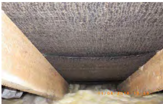
Figure 6.46 Clear eaves area in loft space
