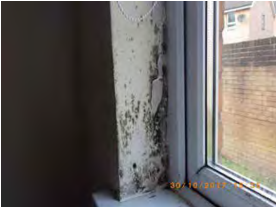
Figure 7.12 Condensation
