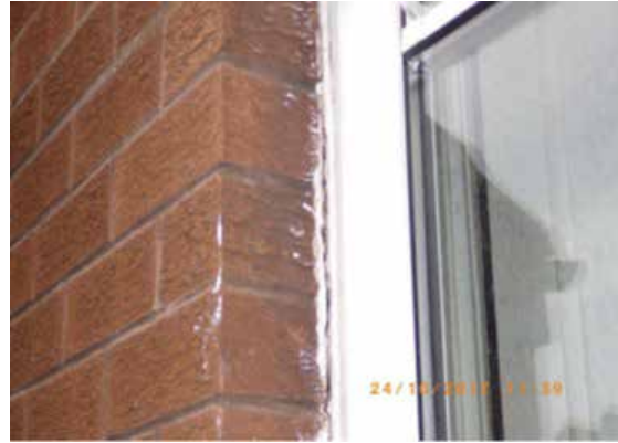
Figure 6.20 Perimeter seals (window)
