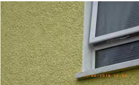
Figure 6.40 Window reveal juncture in a good condition
