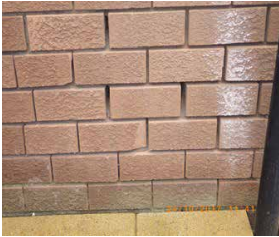
Figure 7.29 Compromised mortar
