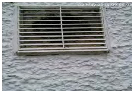
Figure 4.6 Combustion vent
