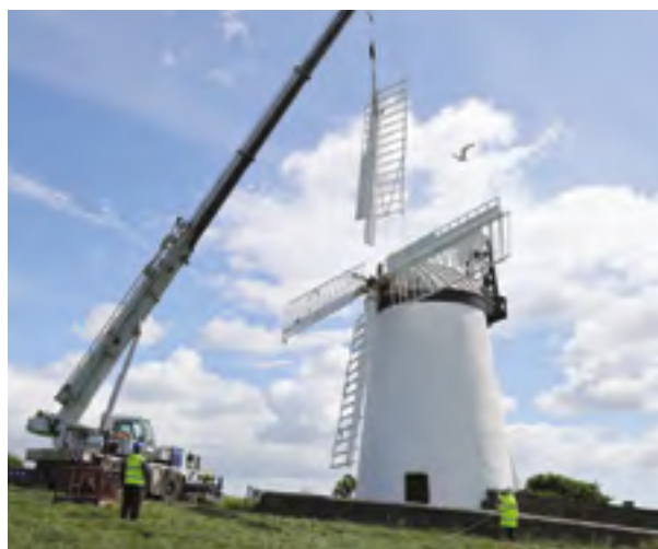
Replacing a sail of the Ballycopeland Windmill, Co. Down, Photo: HED
