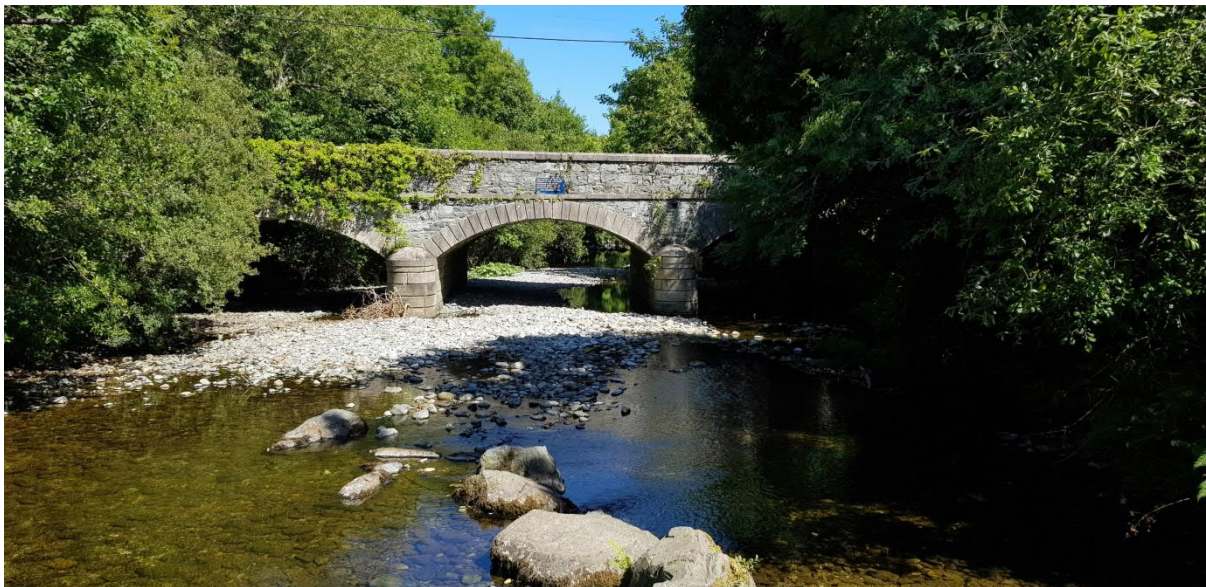
Plate 2: Shimna River where it flows under Bryansford Road. Water levels were low during survey. Broadleaved semi-natural woodland fringes the river.
