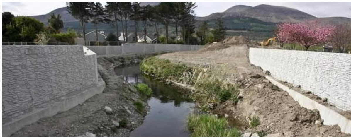
Plate 13.4: Construction of the Burren River Flood Alleviation Scheme
