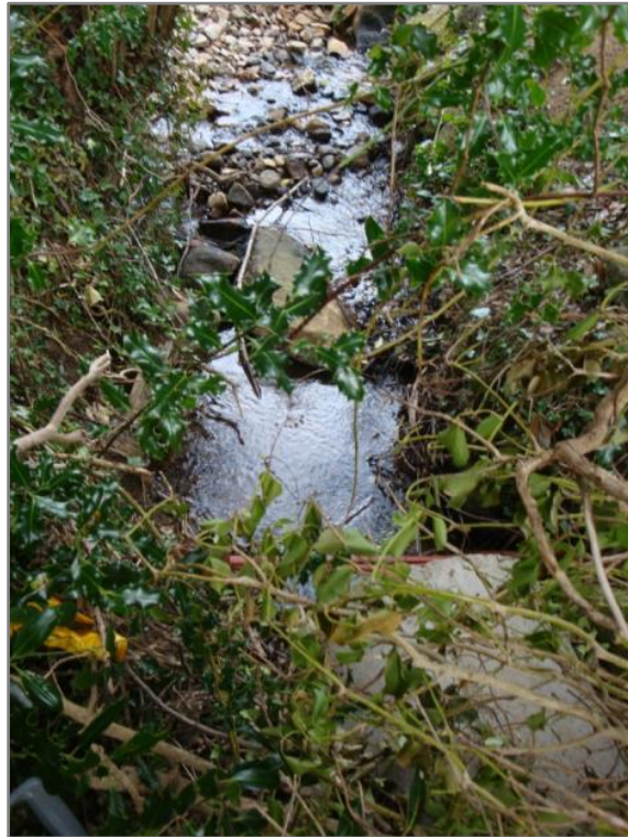
Figure 5.8 Watercourse upstream of 34 Greenan Road
