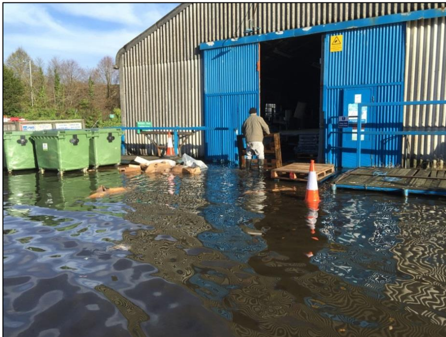
Figure 5.6 Flooding at PWS, Greenbank Industrial Estate
