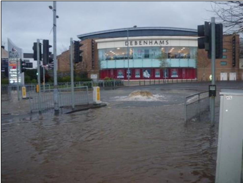
Figure 6.1 Surcharge of NI Water storm sewer at Quays Car Park entry, Bridge Street (November 2014)
