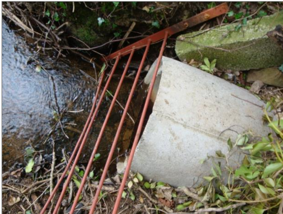
Figure 5.9 Culvert inlet to rear of 34 Greenan Road
