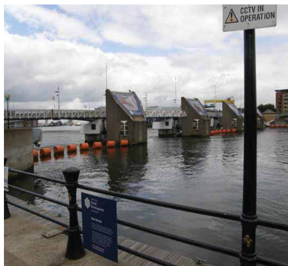
Plate 1.1 – Lagan Weir, which regulates water level within the impounded River Lagan.
