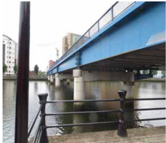
Plate 4.1 – Lagan Railway Bridge crossing the downstream section of the Impoundment.
