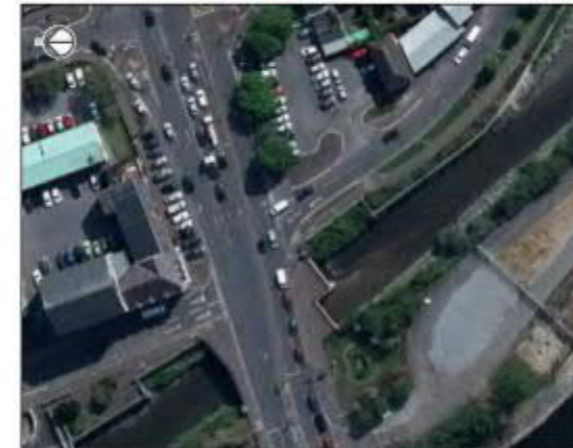
A28 WILLIAM STREET / RIVER STREET
