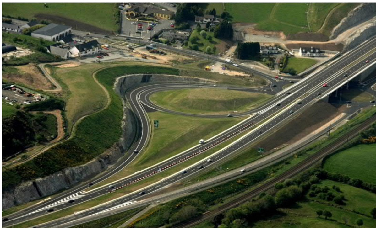
Figure 2.2.1 Cloghogue Roundabout junction southern merge/diverge arrangements
