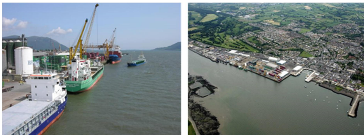
Figure 2.8.1 Cargo handling and Aerial Photography of Warrenpoint Port
