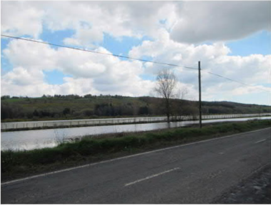
Plate 5.3.9 Section of the Newry Canal (DOW/ARM 029:500)
