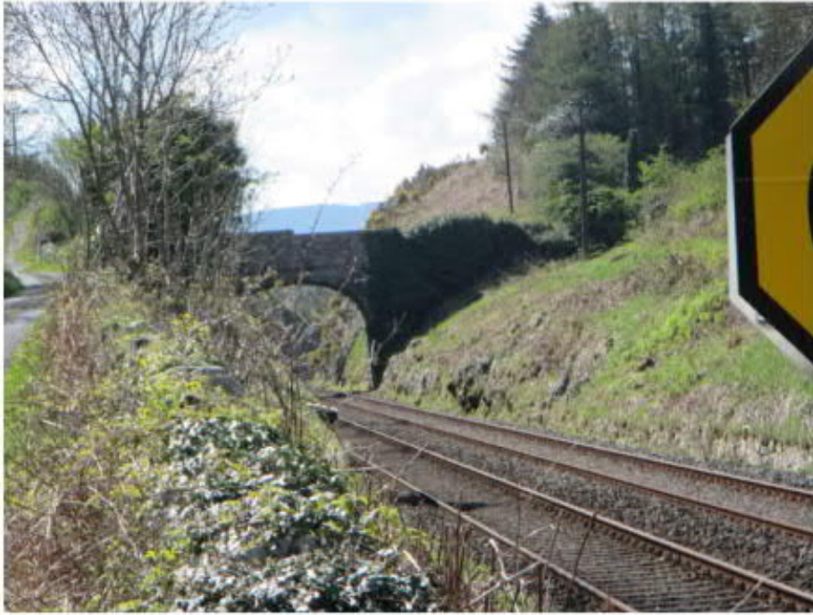
Plate 5.3.5 Bridge (HB16/13/013) carrying Barracric Road over the railway
