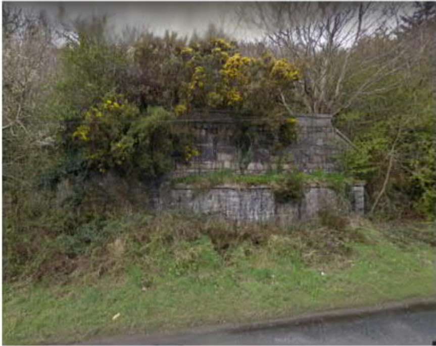
Plate 5.3.7 Remains of railway bridge (00538:006:00)
