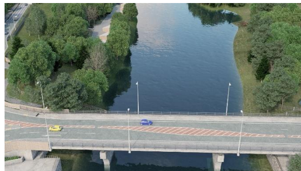
Figure 9 Removal of overhead cables at Erne Bridge
