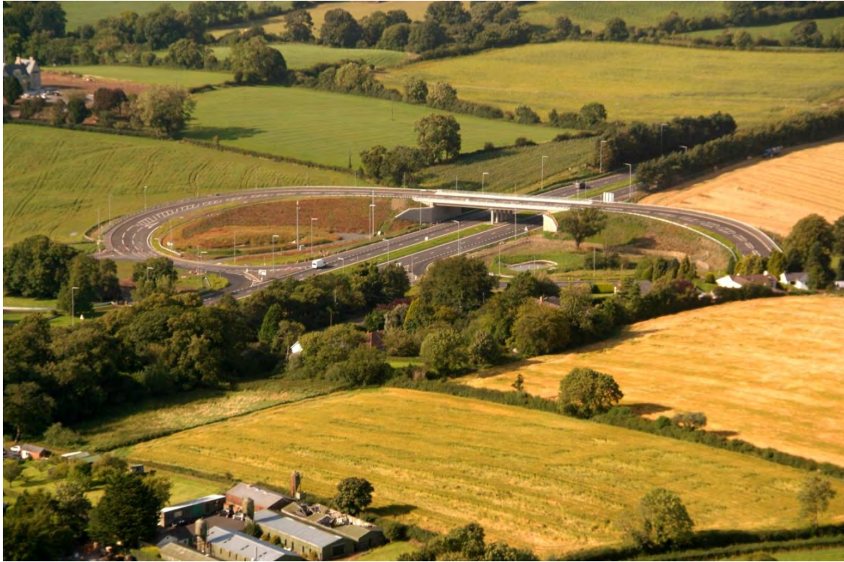
Figure 2.7 Existing Compact Grade Separated Junction on A1 at Hillsborough
