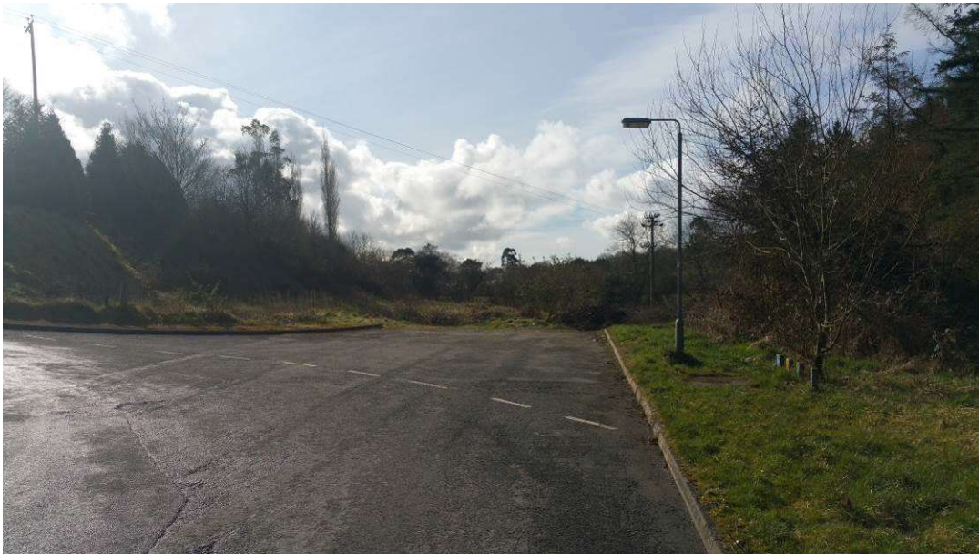
Figure 5.4 – Looking south towards Hamiltonsbawn Industrial Estate from Linsey's Heights (Large groups of trees present, approx. Ch2150m)
