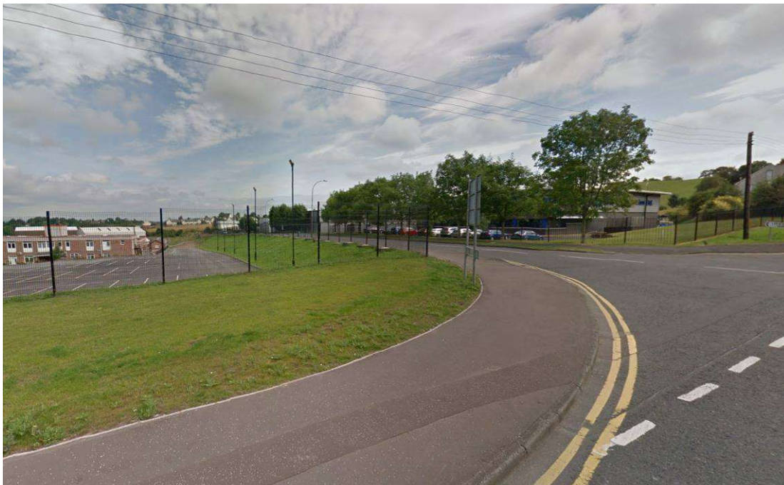
Figure 3.20 – A51 Hamiltonsbawn Road Industrial Estate Access Embankment
