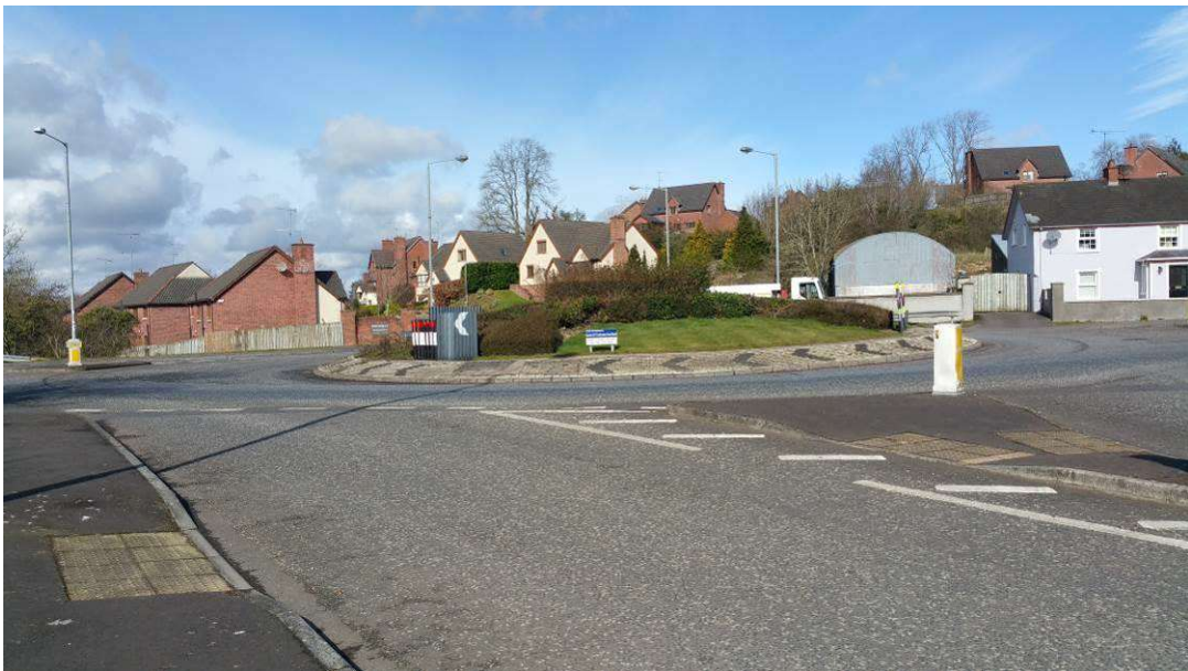
Figure 5.11 – Looking towards the existing roundabout at Drumman Heights / Drummanmore Road (northern tie in)
