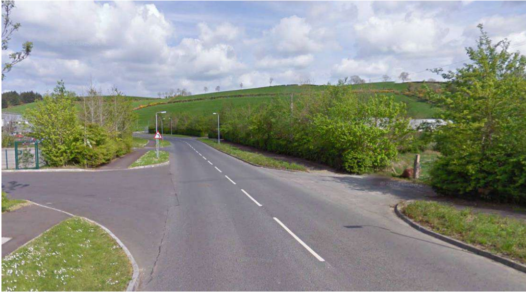
Figure 5.6 – Looking northeast along Edenaveys Road (approx. Ch50m)
