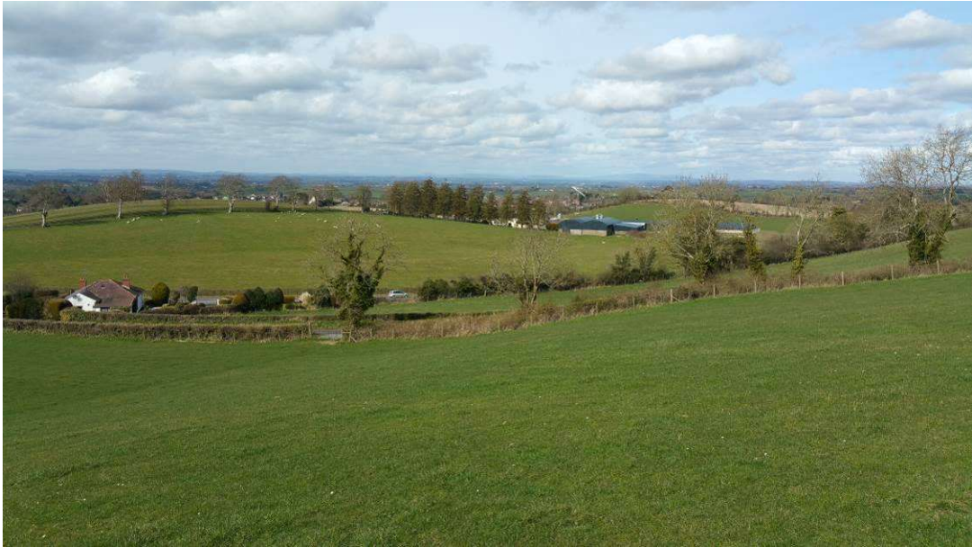
Figure 5.13 – Looking northeast along the line of Option 50 towards the A51 Hamiltonsbawn Road and proposed junction (approx. Ch1650m)
