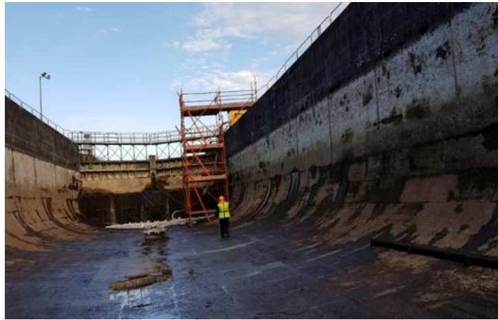
Victoria Lock dewatered
