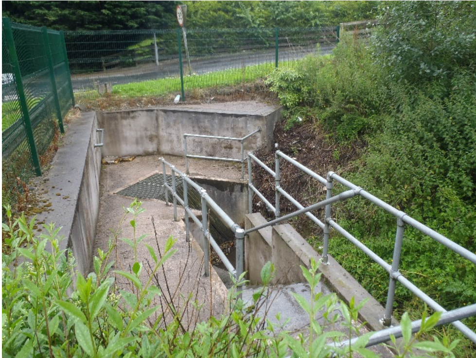
Figure 5-17 - Large concrete watercourse crossing structure at A3 Portadown Road (KDC01)
