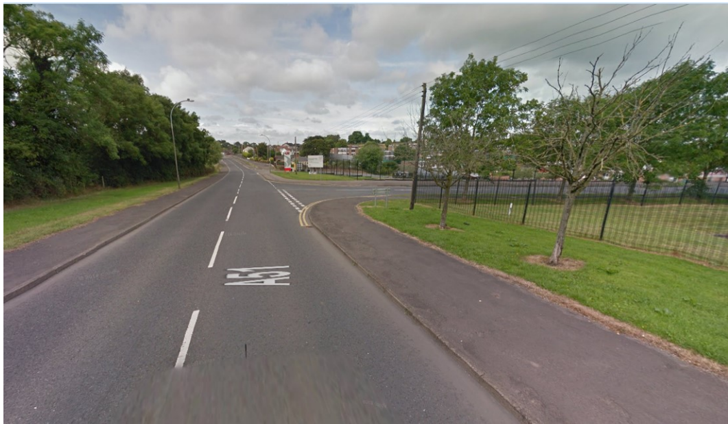
Figure 2-4 - Photograph of the existing A51 Hamiltonsbawn Road at Hamiltonsbawn Road Industrial Estate Junction (looking west towards Armagh City)
