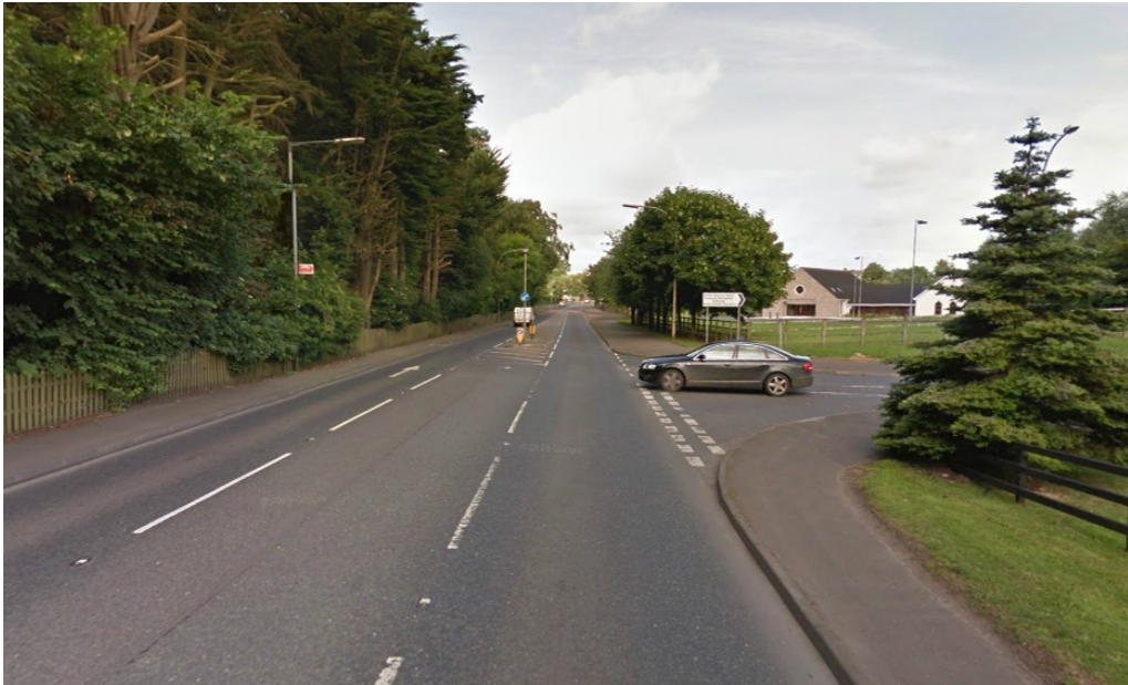
Figure 2-2 - Photograph of the existing A28 Markethill Road at Ardmore Road Junction (looking northwest towards Armagh City)
