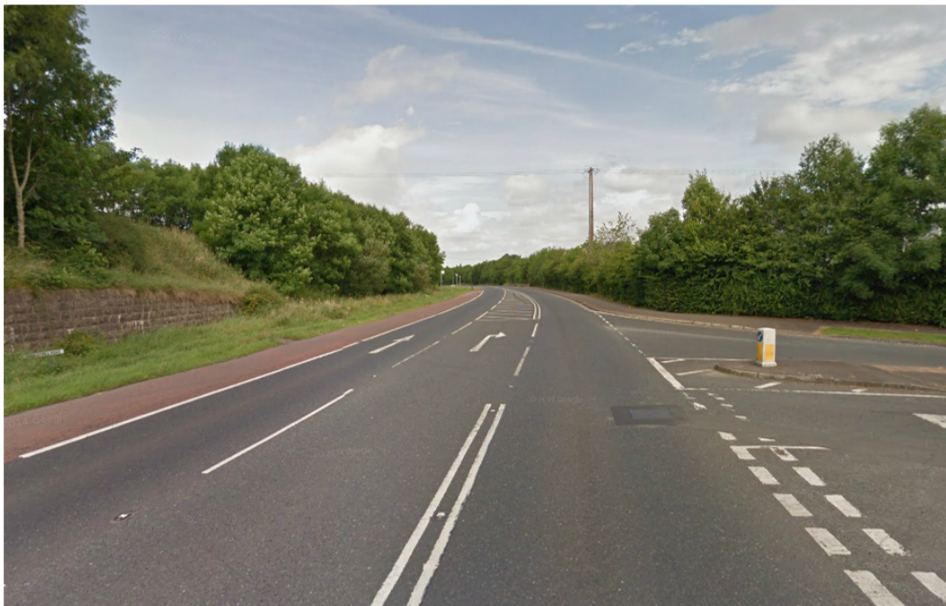
Figure 2-3 - Photograph of the existing A28 Markethill Road at Edenaveys Industrial Estate Junction (looking northwest towards Armagh City)
