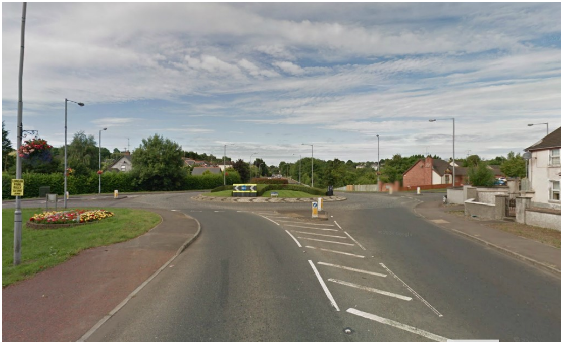
Figure 2-7 - Photograph of the existing roundabout linking the A3 Portadown Road with the housing estates at Killuney Road and Drumman Heights (looking west towards Armagh City)
