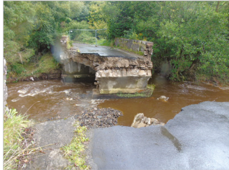
Glenrandal Bridge, Claudy
