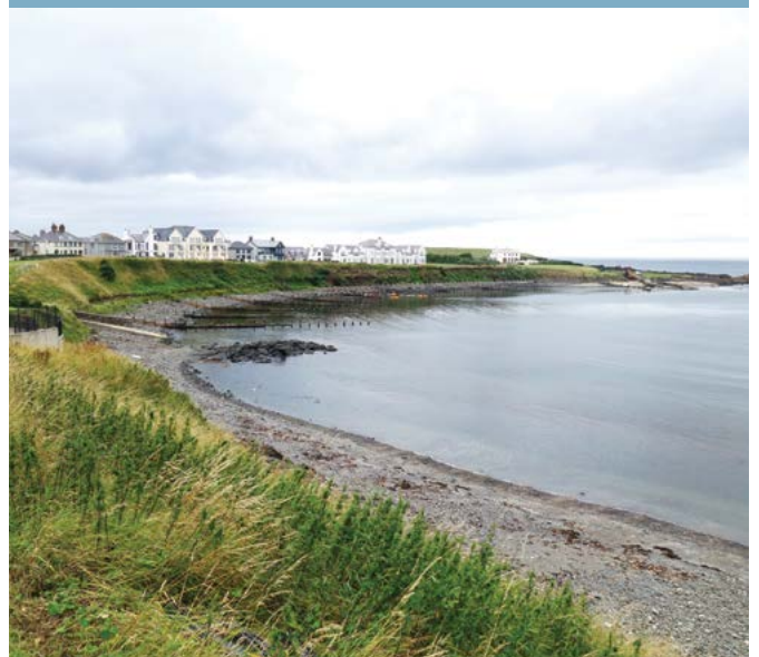
Photograph 5. Piers at Portballintrae that have resulted in beach erosion
