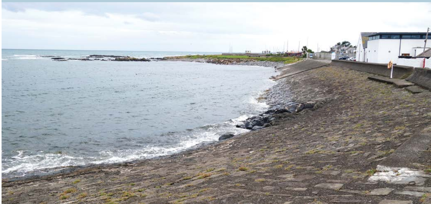
Photograph 9. Stone revetment in Donaghadee
