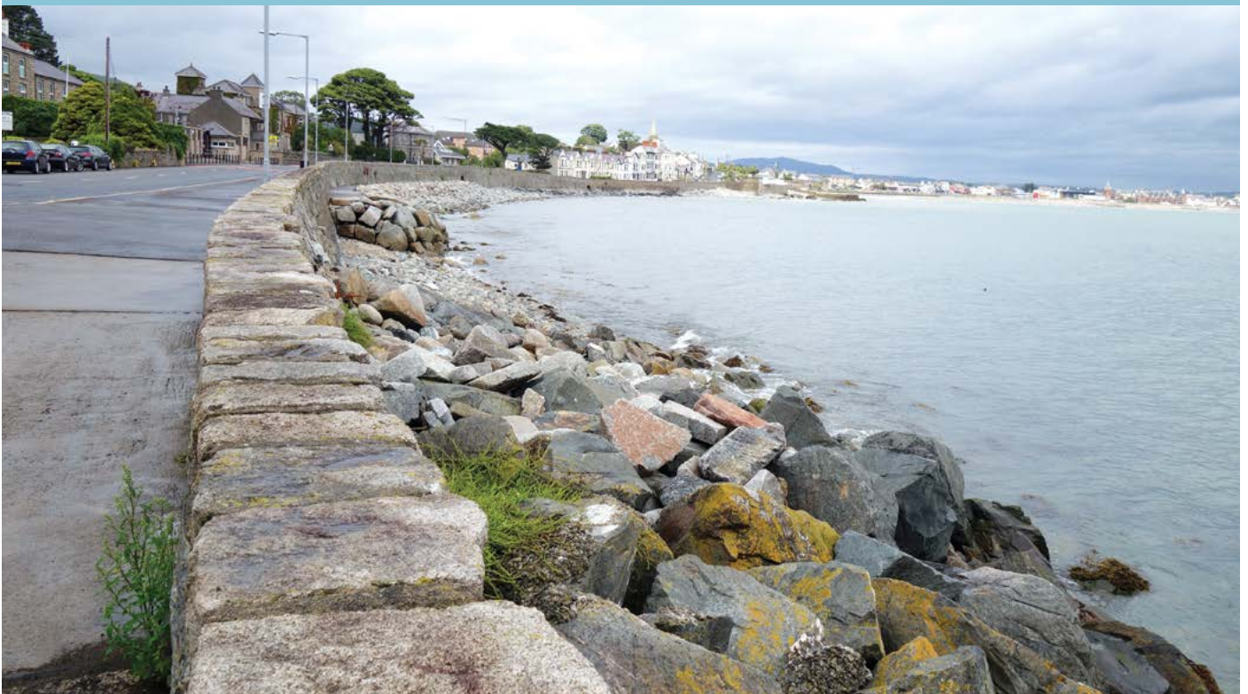
Photograph 1. Coastal Protection at Newcastle, County Down
