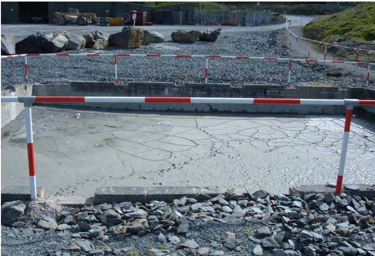
Settlement pond to trap silt
