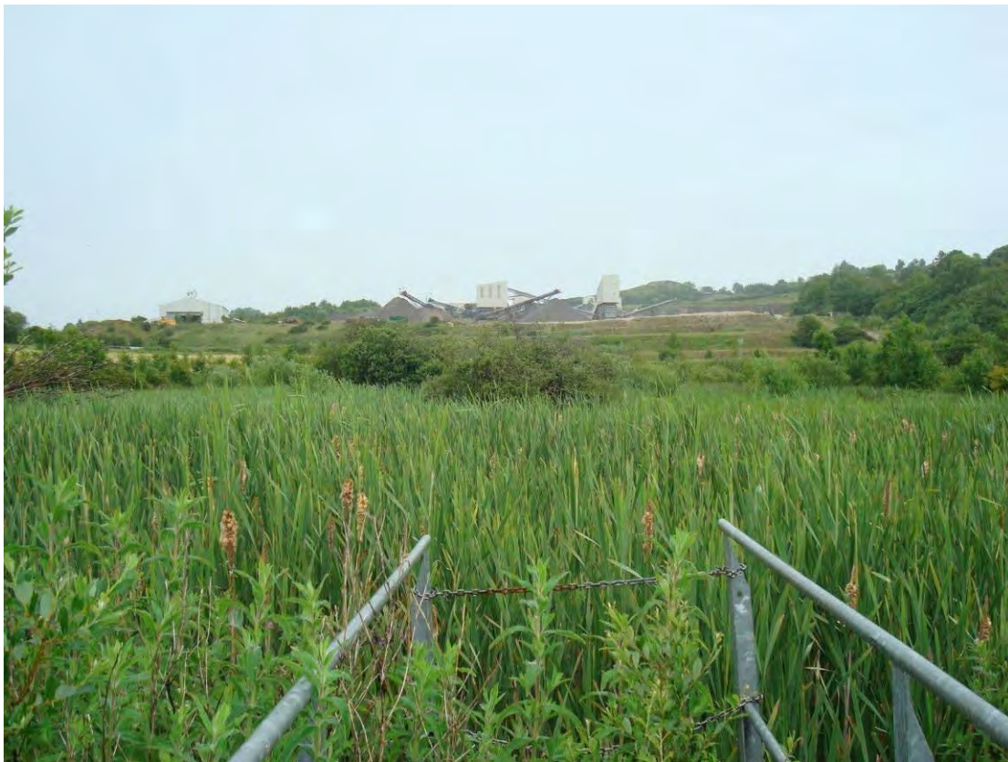
The density of reed growth and native species such as willow shrub benefits biodiversity as well as treatment of water prior to discharge in the series of settlement ponds at Doon Quarry, Co Fermanagh.
