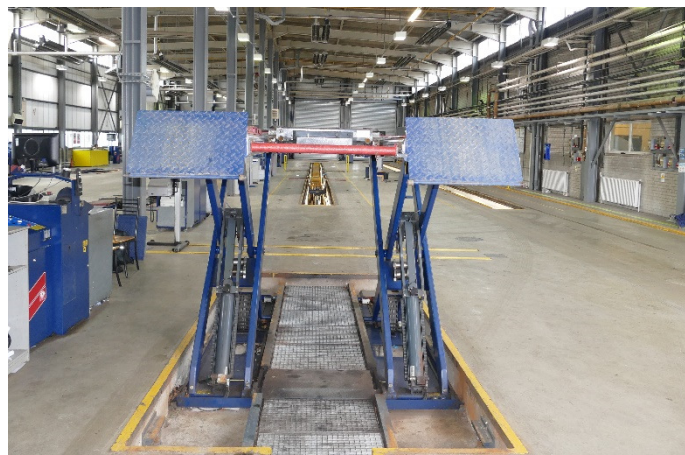
Elevation looking from exit end towards entrance
