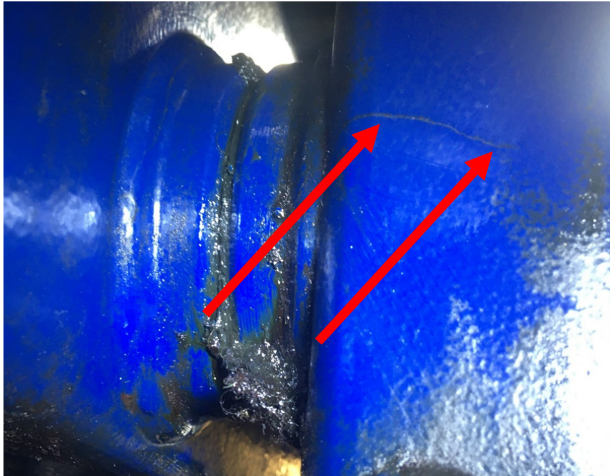
Cracking observed to underside of box section
