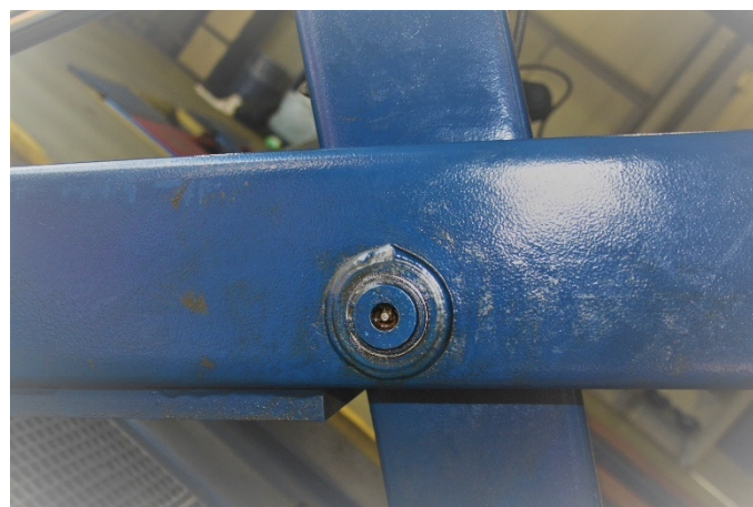
Typical outer box section – outside face
