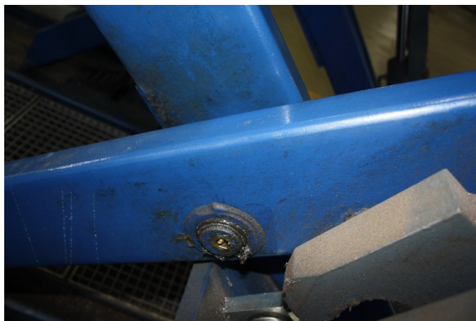
Typical inner box section – outside face
