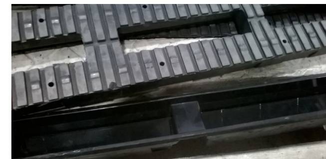
Figure 20b: It also can be fitted with flaps which are designed to allow slurry to drop into the tank but reduce fresh air contact with slurry in the tank to minimise ammonia losses.
