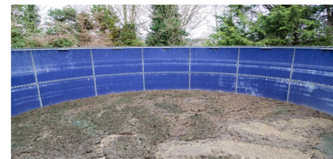
Figure 10: Slurry tank with crust which can help to prevent ammonia loss.
