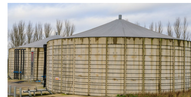
Figure 6: Fixed cover on an above-ground concrete slurry store at CAFRE.
