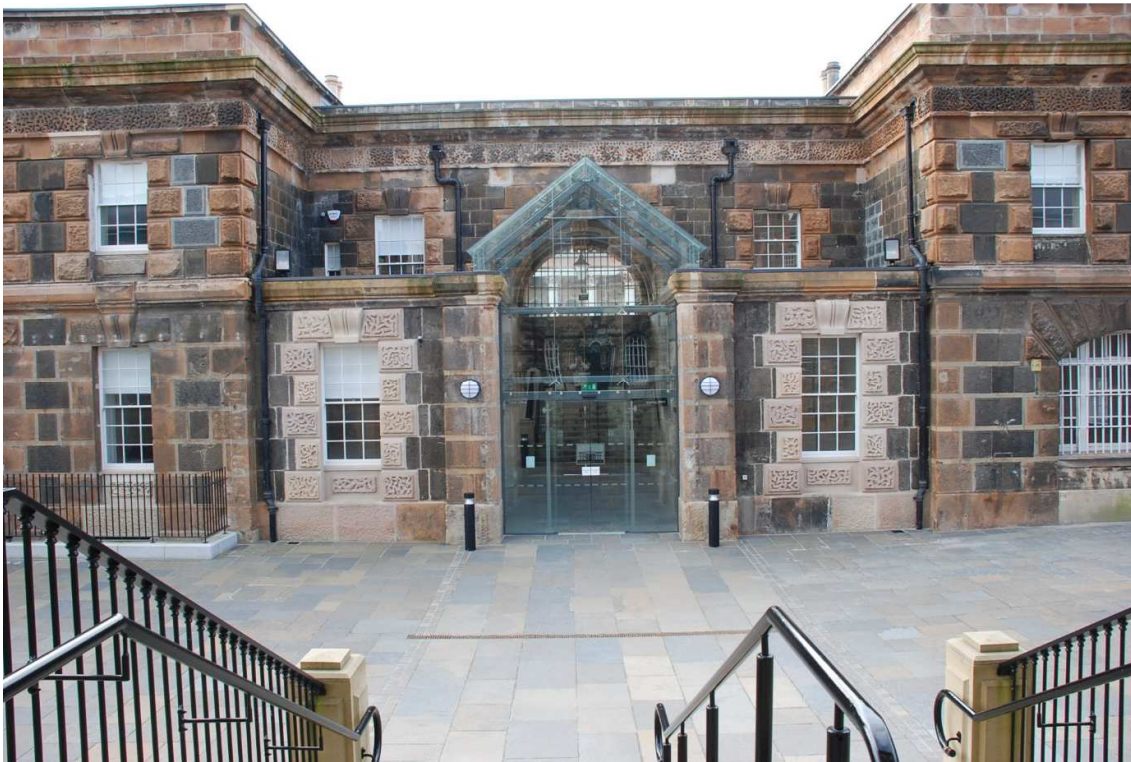
Crumlin Road Gaol (HED)
