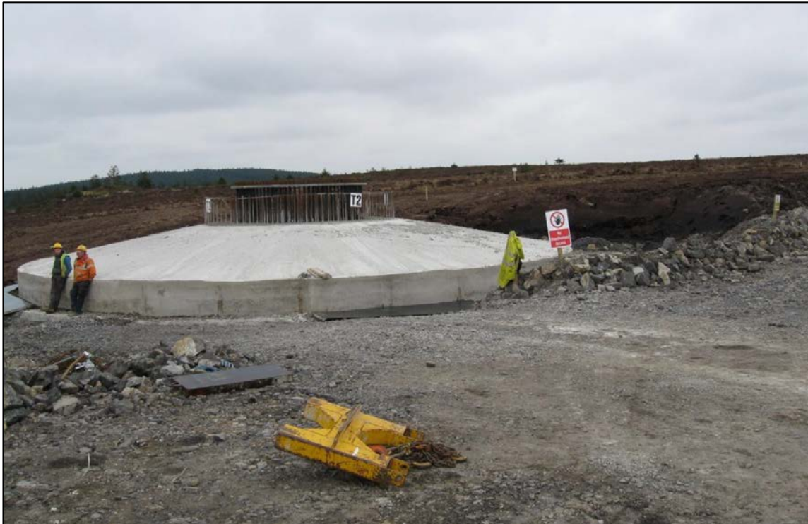
Figure 1: Construction of the foundation of a single wind turbine.
